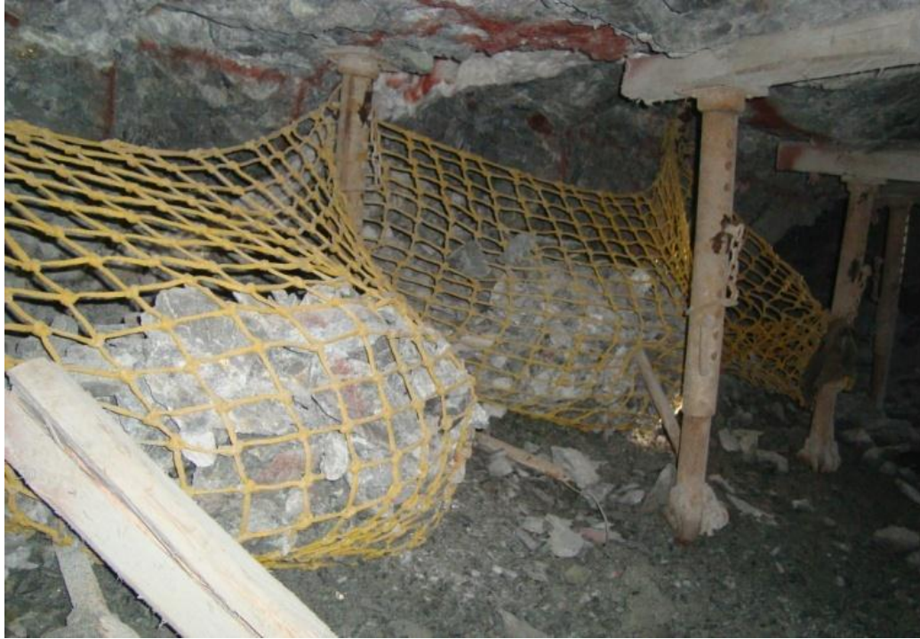
Figure 6.3.2 In-stope netting used on the face at Thuthukani Shaft, KDC. (Source: Personal Collection)
