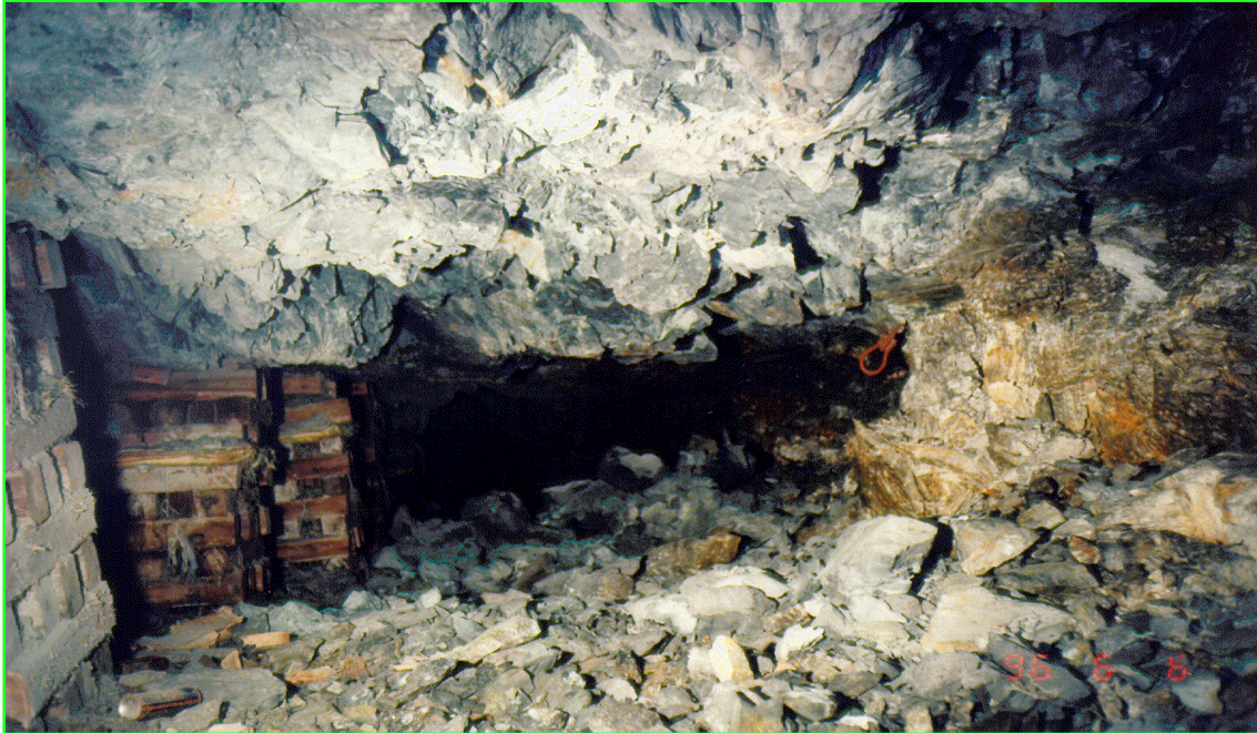
Figure 5.5.2 Panel with no Pre-conditioning conducted. (Source: Toper, 2003)
