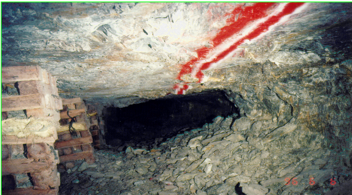
Figure 5.5.3 Panel with Pre-conditioning conducted. (Source: Toper, 2003)
