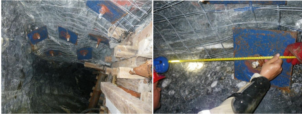
Figure 7.6.1 Rock consolidation at Thuthukani Shaft, KDC.
