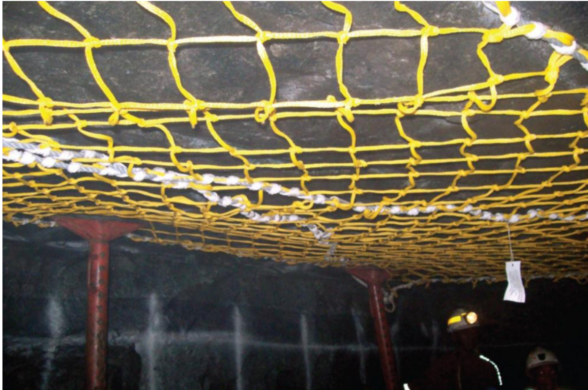
Figure 6.2.2 Typical installation of in-stope netting.
