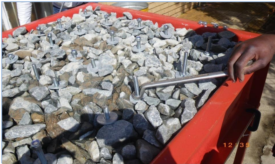
Figure 7.2.5 Tightening the bolts. (Source: Gold Fields, 2012)
