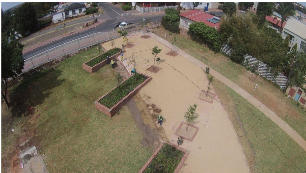
Figure 14: Westdene Dam Redevelopment, Johannesburg
