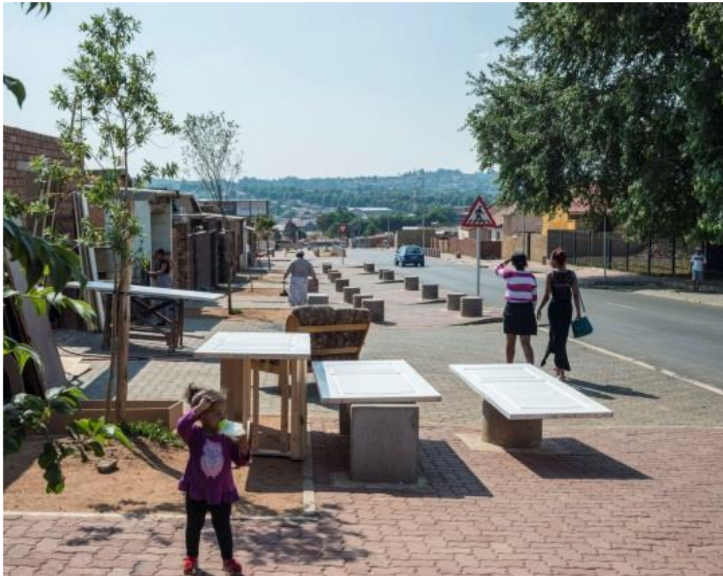
Figure 13: Widened pavements in Westbury, Johannesburg
