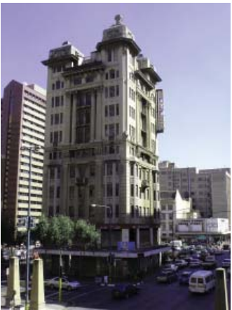
The vacant Palace site with the Barbican building
