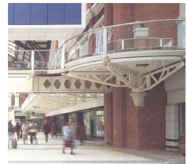
New walkway 'clipped' onto an old wall of the station. (Derbyshire 1991: 106)
