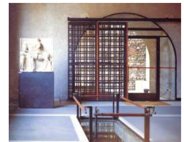
Steel door positioned over an entrance door. (Los 1993: 80)
