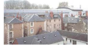
The grey barrel roof of the centre blends in with the slate pitched roofs of the neighbouring houses. (Di Battista 1994: 10)
