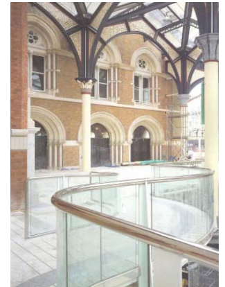
The glass balustrade in foreground with replicated arches in background. (Derbyshire 1991: 107)
