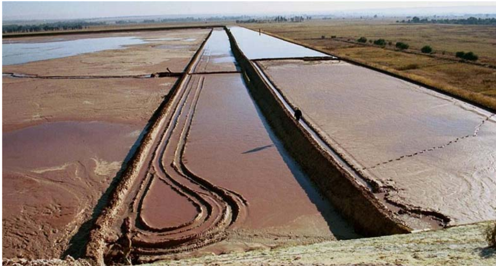
Figure A.1: Modern paddock construction, note the two day walls (Robinson, 2010)
