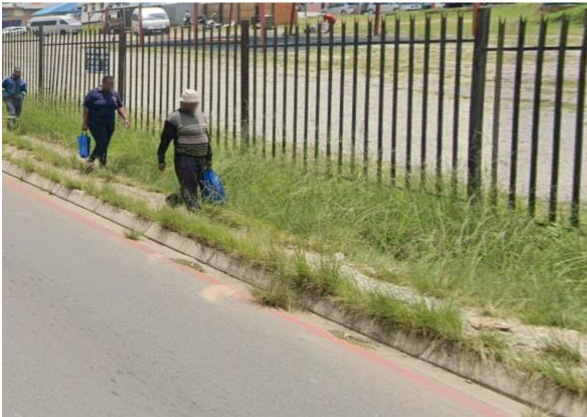
Figure 4.3: Unmaintained walkways within the study area.
