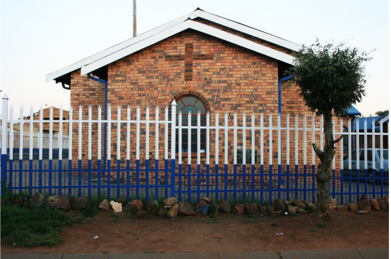
Figure 15: Apostolic Church, Mapetla.
