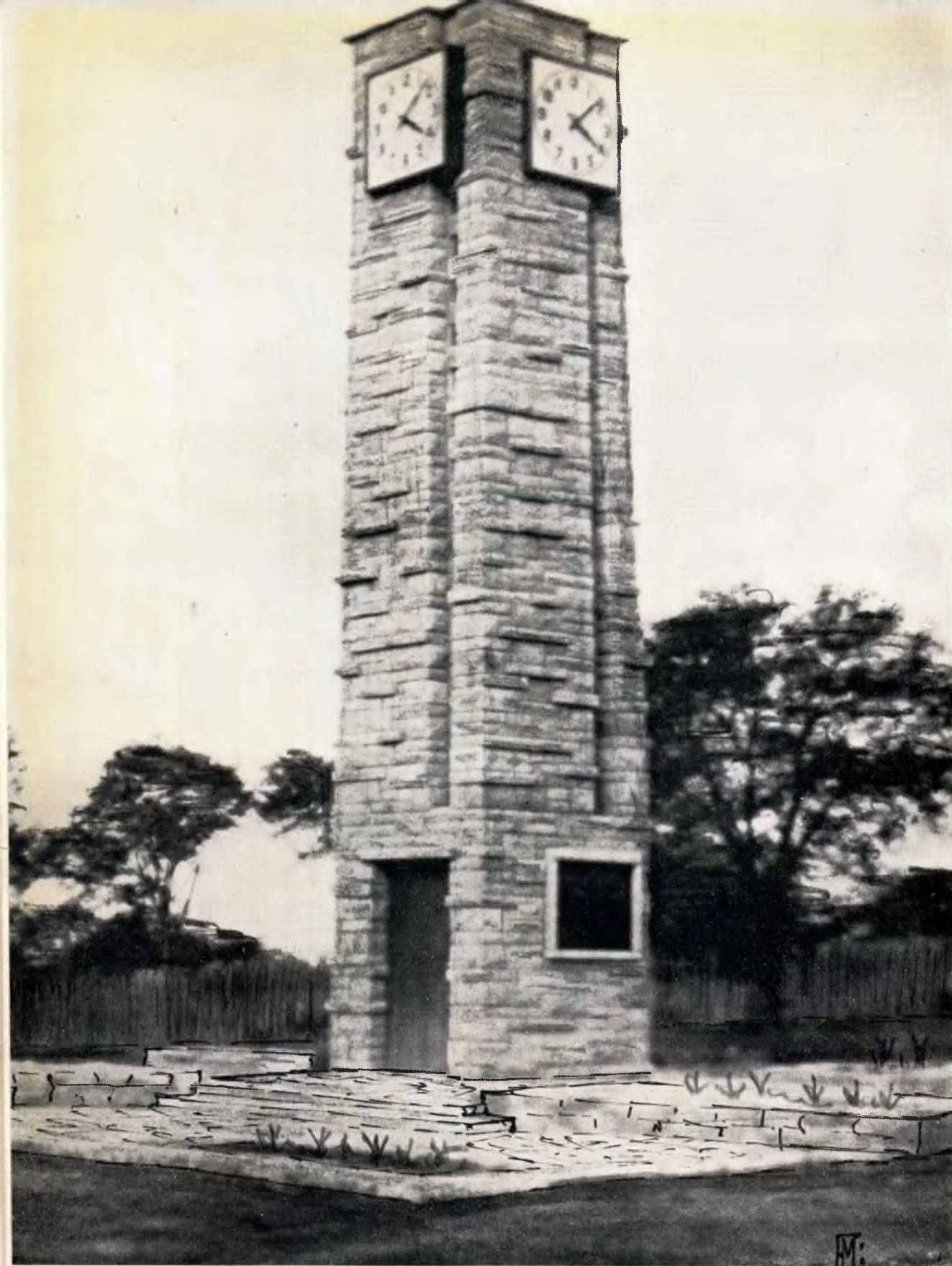
PAPENFUS MEMORIAL CLOCK fitted with turret type movement with four dials operating from one movement. Complete with bell (Note "G" 140 lbs. weight). Installed to specification by the Architects by Greaves (Pty.), Ltd. (Wholesale), Distributors for Smith's Electric Clocks, Johannesburg, Durban, Cape Town.
