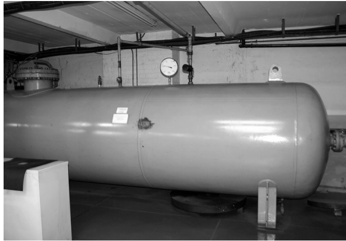
Figure 4.3: Supersonic wind tunnel storage vessel
