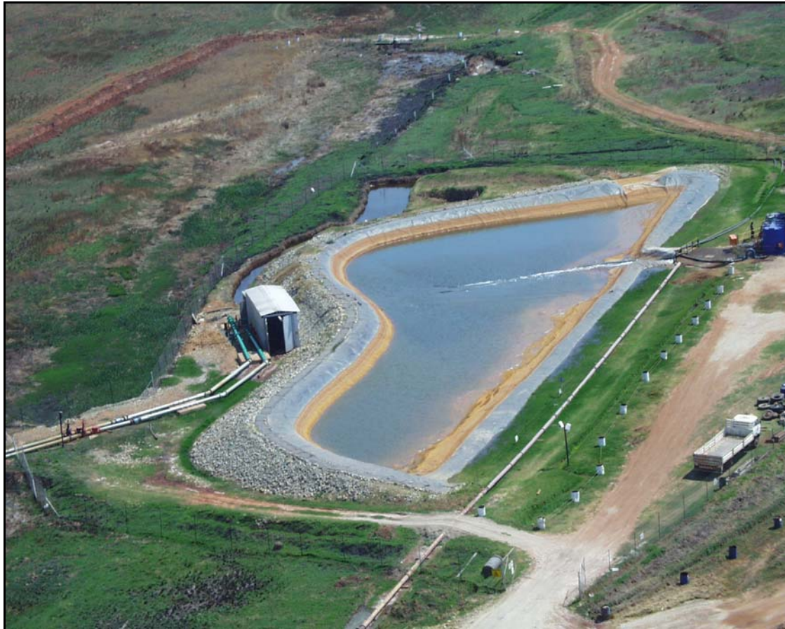
Photo 2 – The dam constructed to intercept water decanting from the underground mine void.
