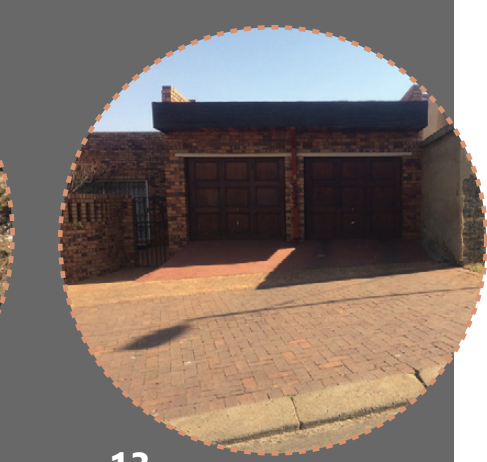
13 RESIDENTIAL AREAS SURROUND THE SITE ON THE WEST AND EAST
