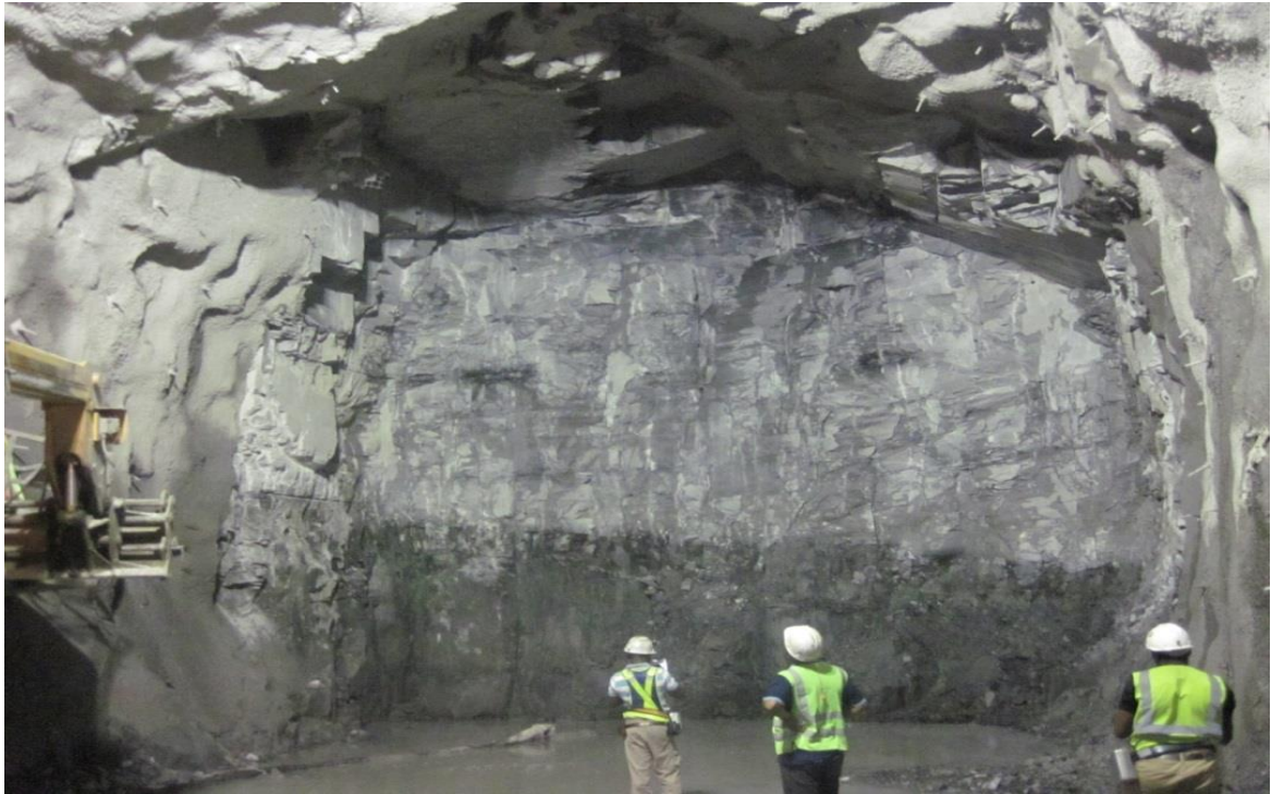
Figure 3-6: The face of the tailrace tunnel at chainage 165.60m
