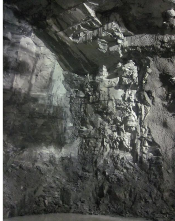
Figure 3-9: Right sidewall of the tailrace tunnel at chainage 165.60m
