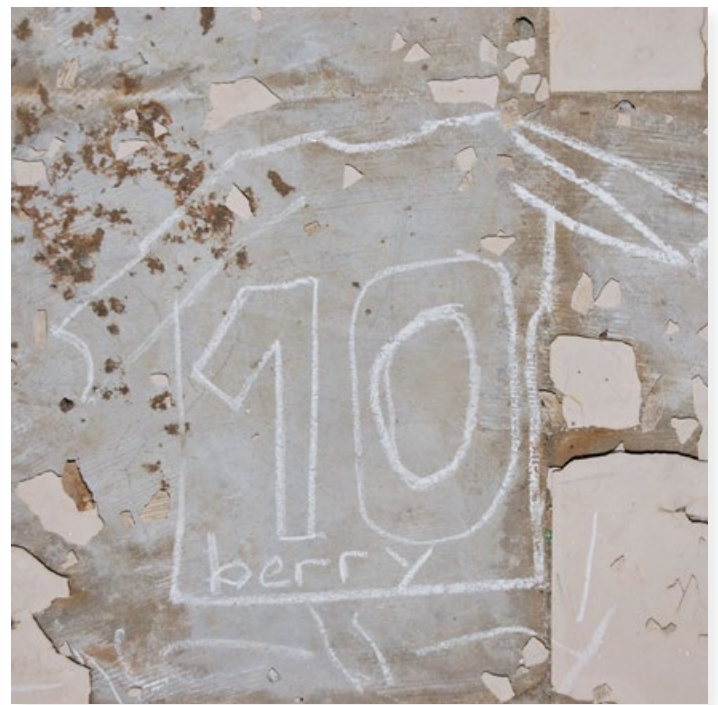
'Berry 10' shirt drawn on slab of demolished school building, Riverside Park, KwaThema, 2011
