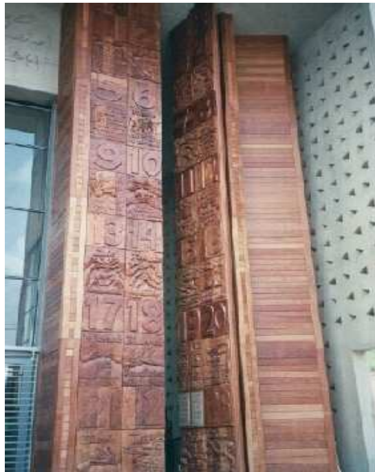
Plate 4.5.7: Doors to the outside of the Constitutional Court.
