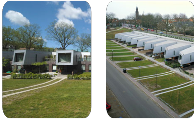
Fig 26 -27. The Soundbarrier Houses (Source: www.archrecord.com )
