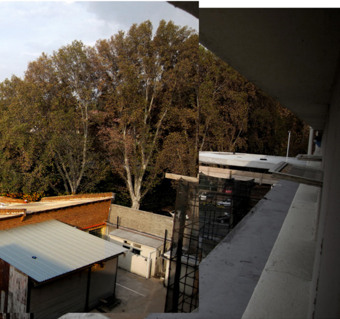
Fig 76. Site photo (Source: author's own)
