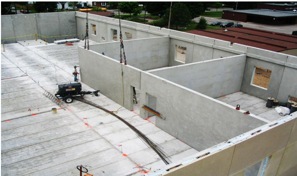
Figure 2.4: Precast wall installation-wall to wall (CPCI 2012)
