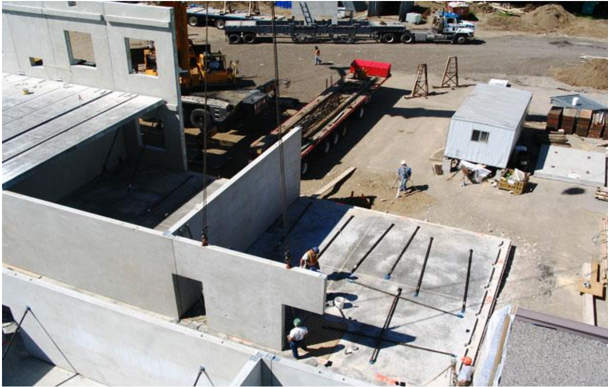
Figure 2.3: Precast wall installation-wall to slab (CPCI 2012)
