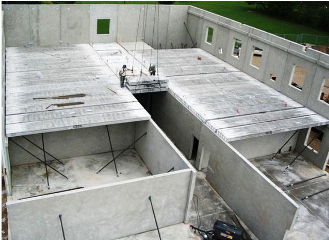
Figure 2.5: Precast concrete slab installation (CPCI 2012)
