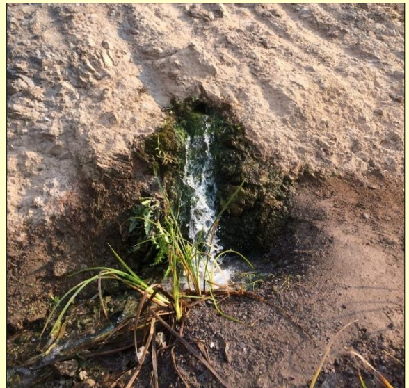
d) Seepage through a horizontal drain hole on the northeastern highwall of Mashi Pit.
