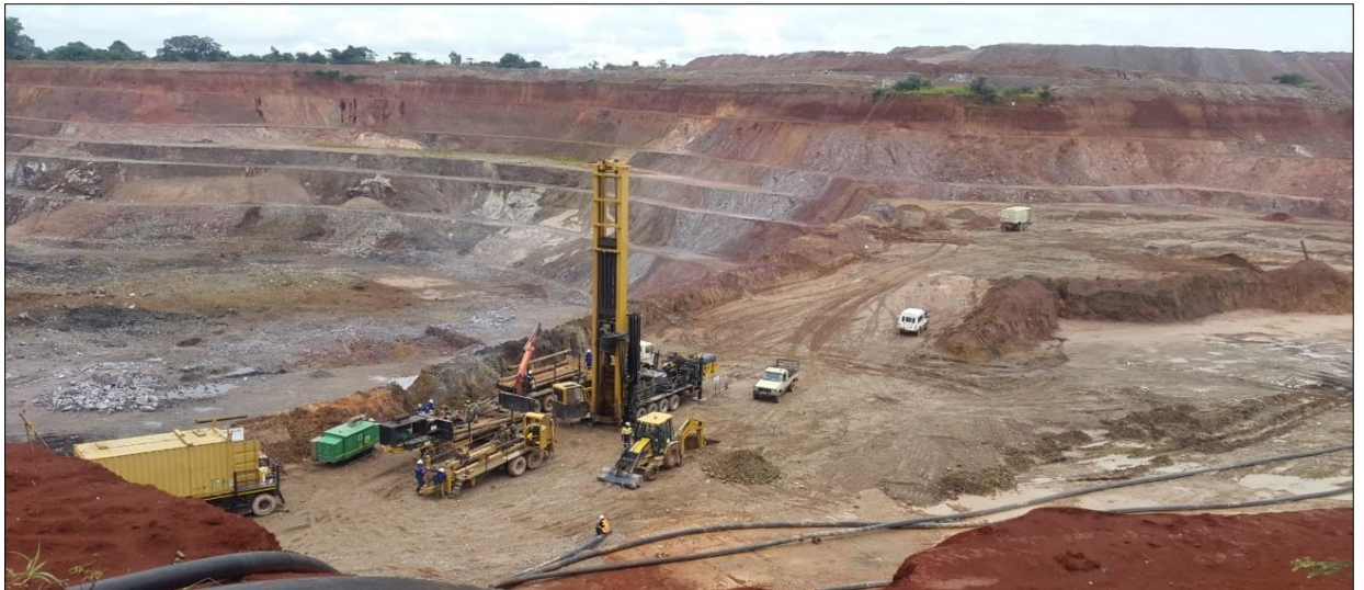
Figure 3-1: Photograph of CSRC rig setup for drilling of a dewatering borehole on the saddle between the Mashi and Central pits saddle.
