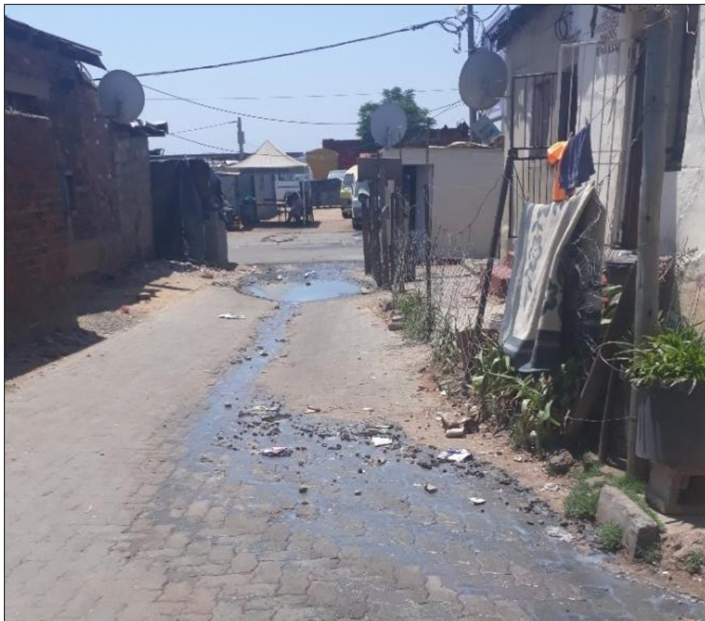
Figure 5.4: Sewage Overflows in RCA
