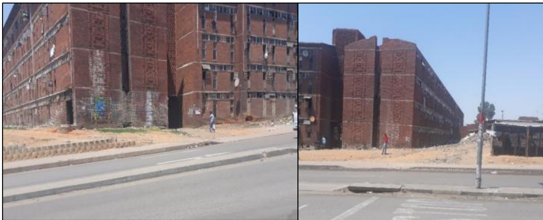
Figure 5.1: Dilapidated Madala (M1) Hostel
