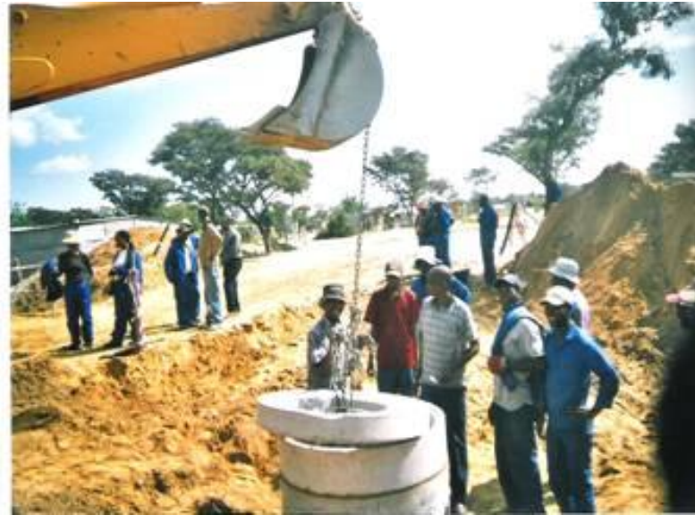
Figure 5.4: The TLB assisting with manhole construction
