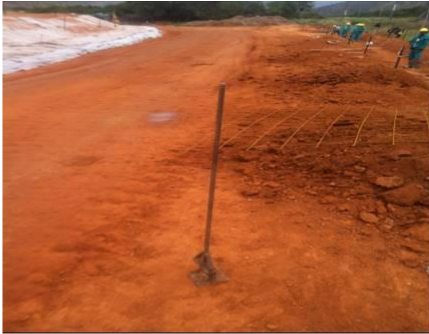
Figure 4.2: Hand-held, locally made steel compactor
