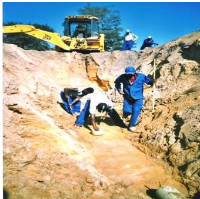
Figure 5.5: Deep excavation at Phagameng Extension 8 using the TLB
