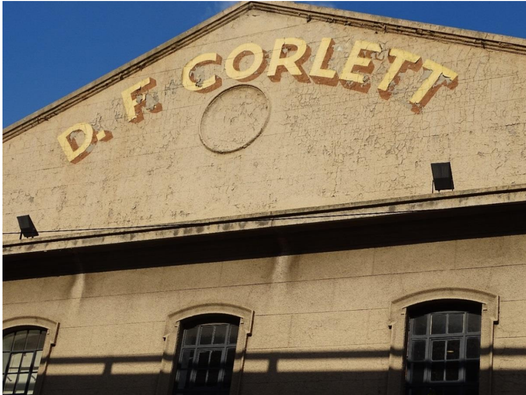
Figure 6.1 The D.F. Corlett Building.
