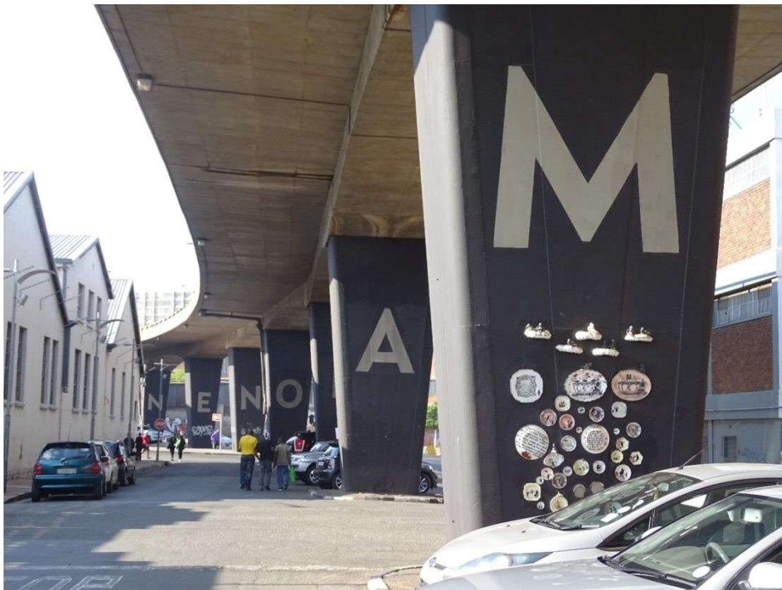
Figure 6.9 The M2 freeway on-ramp, under which displaced people sought shelter.
