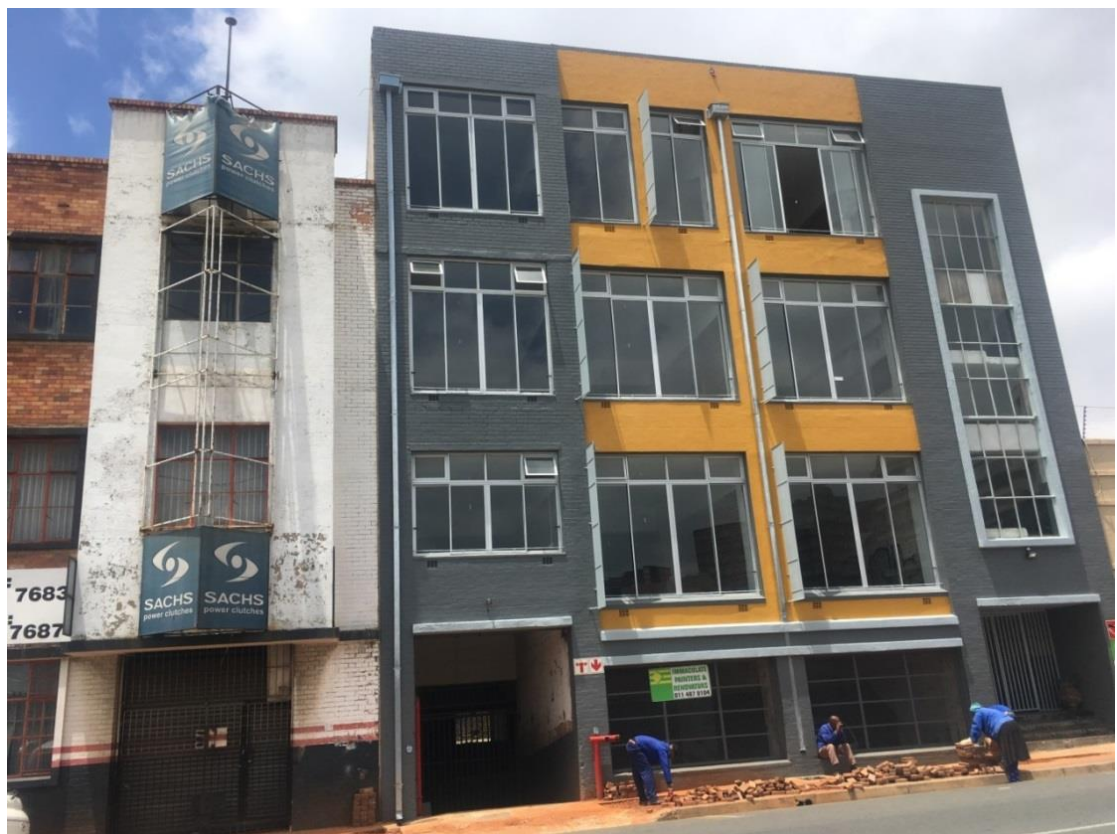
Figure 6.10 The Mainframe Building (the renovated ‘Radiator Centre’ Building).
