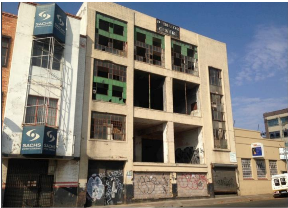
Figure 6.8 The 'Radiator Centre' Building. Source: Mafadi Property Sales (n.d.).
