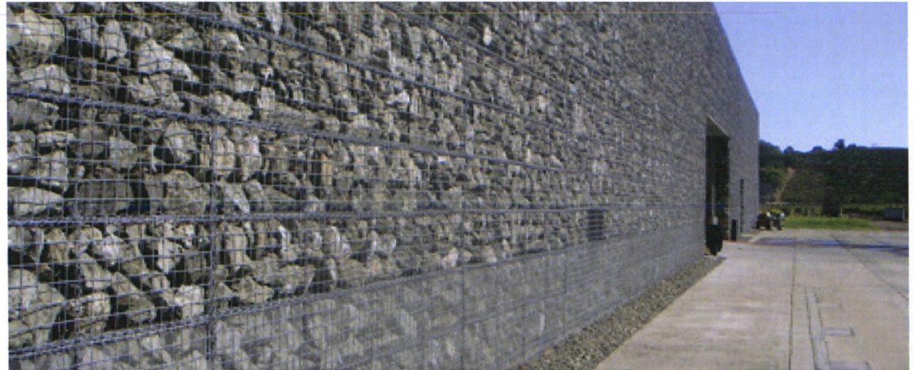
FIG 7.64: Exterior wall view
