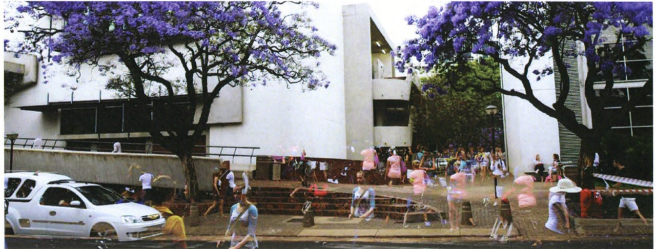
FIG 3.56: University of Pretoria, Centenary building, Pretoria, Photo collage 1
