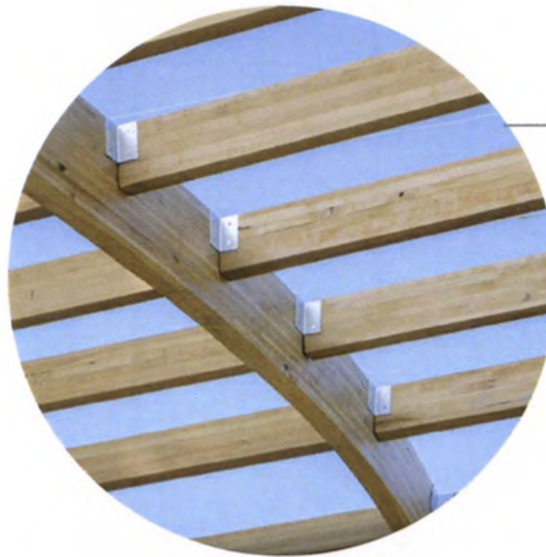
FIG 7.47: Laminated timber pergolas
