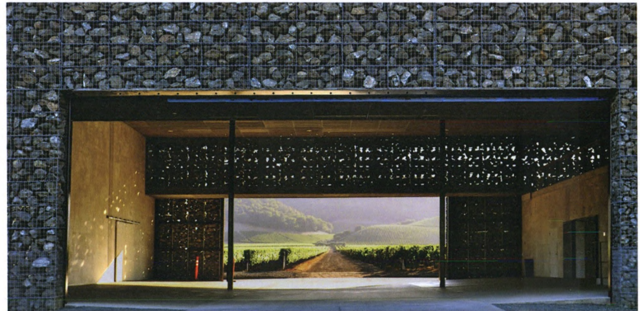
FIG 7.65: Exterior wall view
