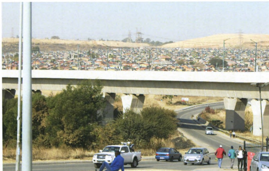
FIG 5.8f: Gautrain flyover bridge.
