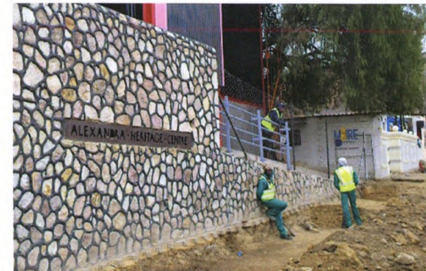
FIG 5.8e : Alexandra Heritage Centre, Peter Rich Architects.
