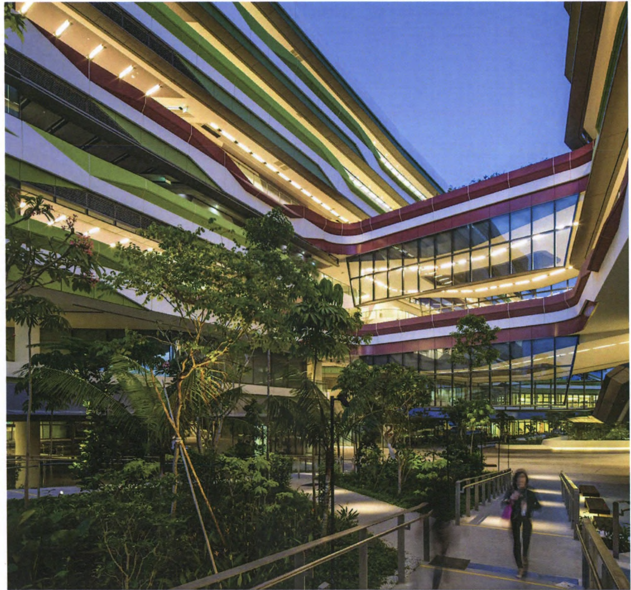
FIG 3.52: Singapore University of Technology and Design ,UNStudio + DP Architects
