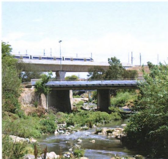
FIG 7.7: Site: View river looking towards Malborow drive and Gautrain flyover.
