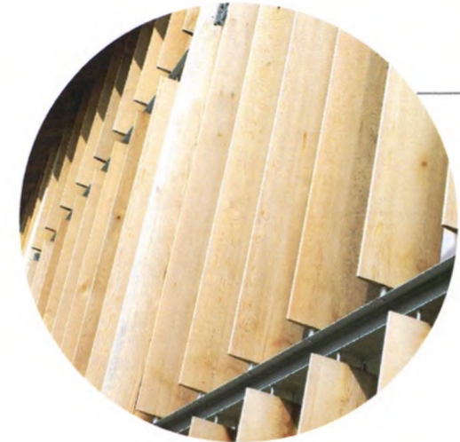
FIG 7.49: Timber facade screens
