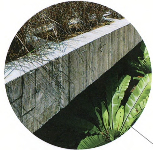
FIG 7.36: Off shutter concrete bridges
