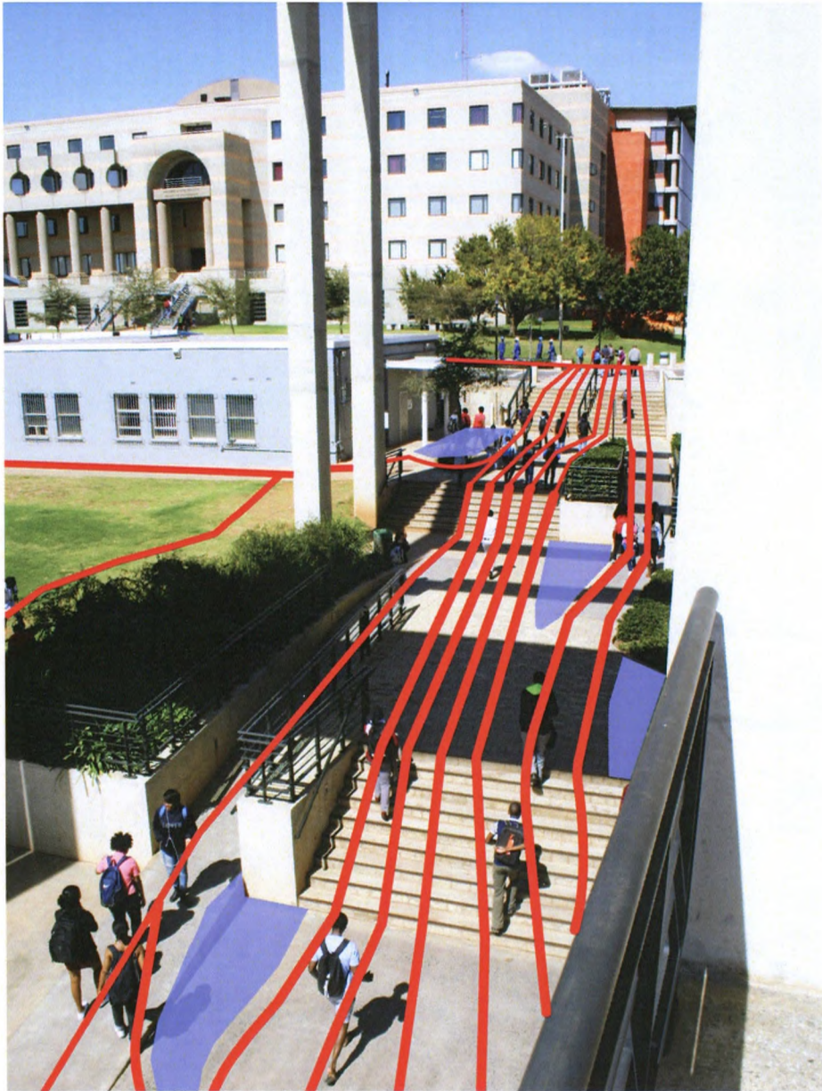
FIG 3.59: Wits University, Science Stadium stairs.
