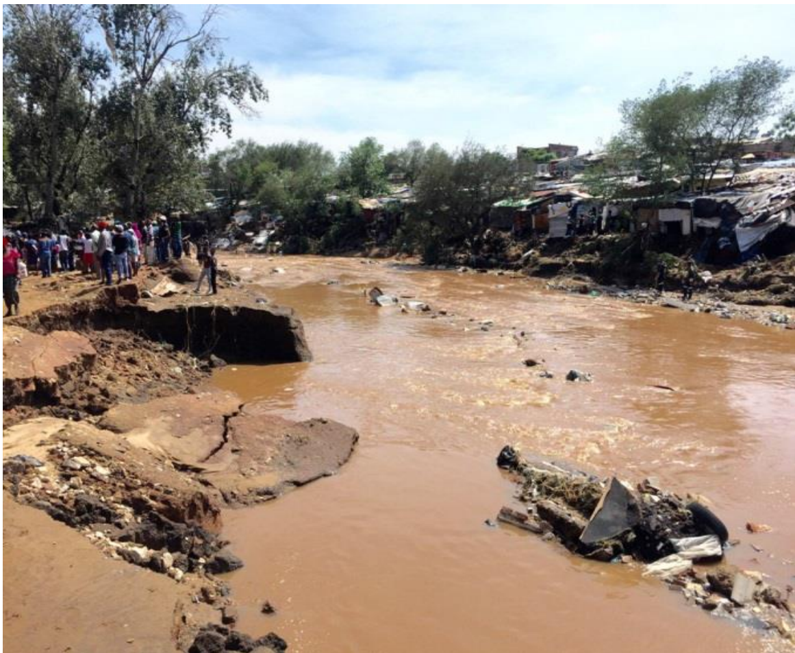
Figure 4.13: The collapsed river bank, Alexandra (Dlangamandla, 2016).
