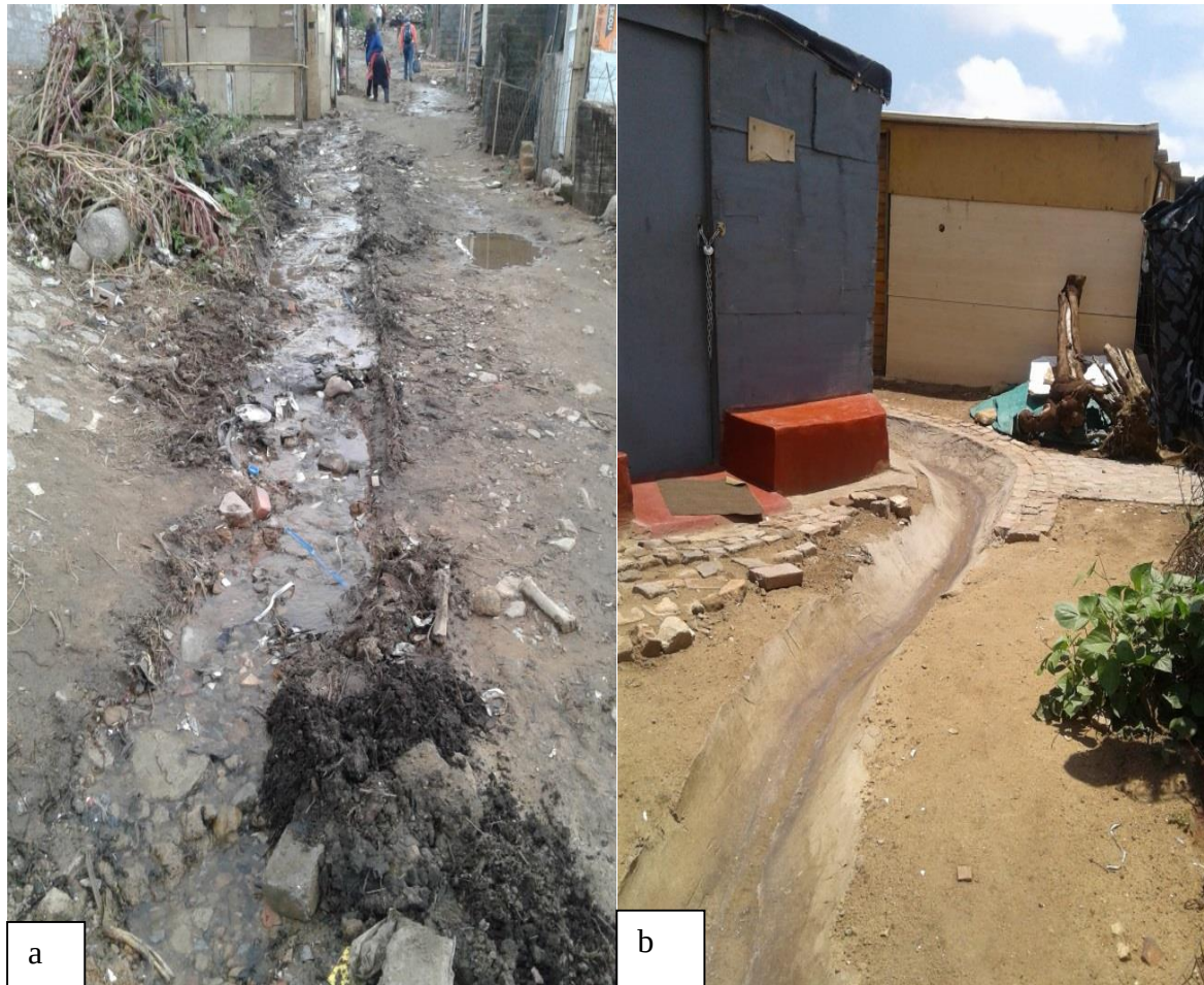
Figure 4.25: Water channel trenches.(a) Not cemented (23/01/2018) and (b) Cemented (23/01/2018).
