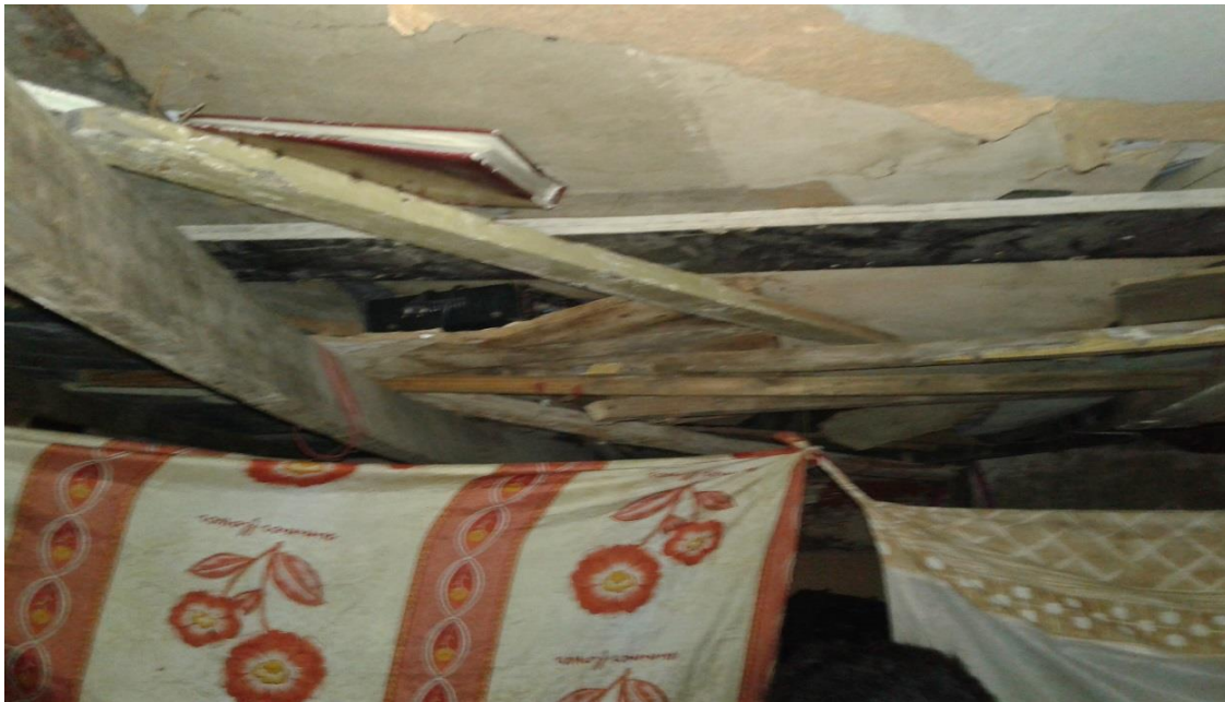
Figure 4.14: Roof from the inside made out of wooden boards (01/03/2018).
