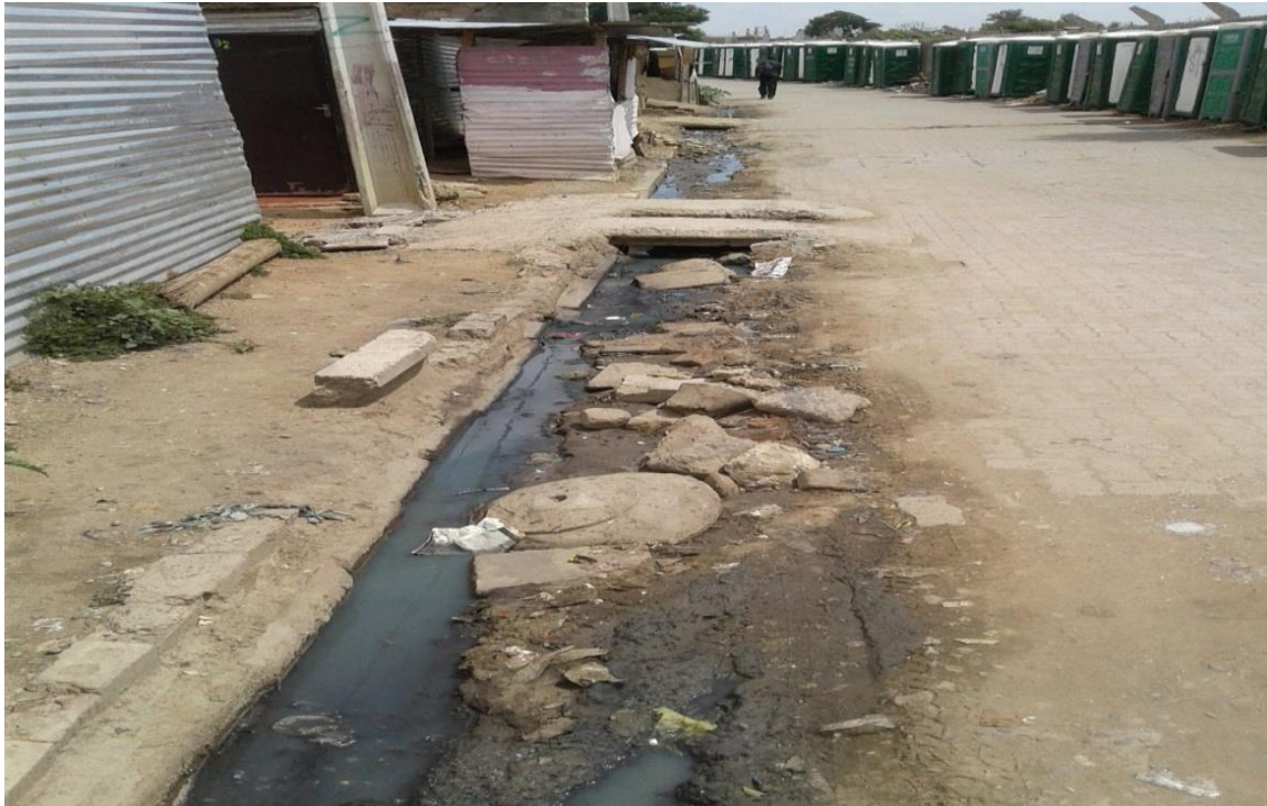
Figure 4.16 Paved road and mobile toilets (23/01/2018).
