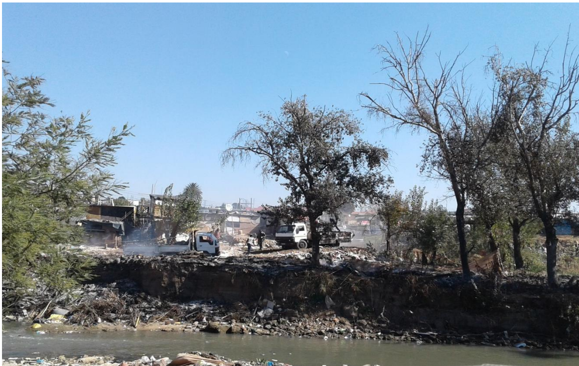
Figure 4.27: Trucks dumping rubble on the Jukskei River banks (07/06/2018).
