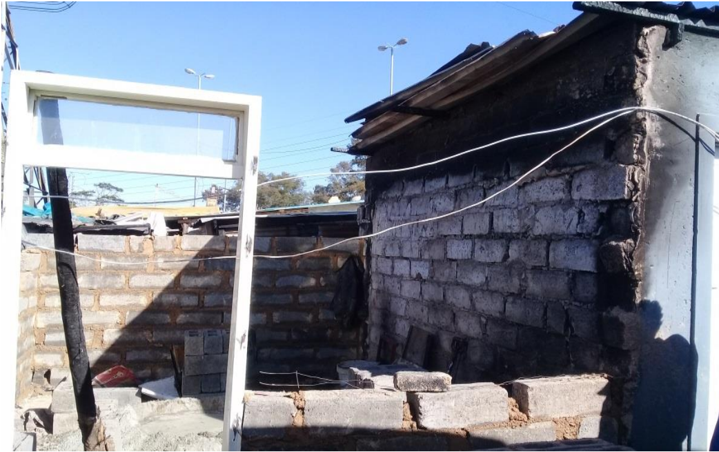
Figure 4.22: Rebuilding with bricks after a shack was burnt down (03/07/2018).
