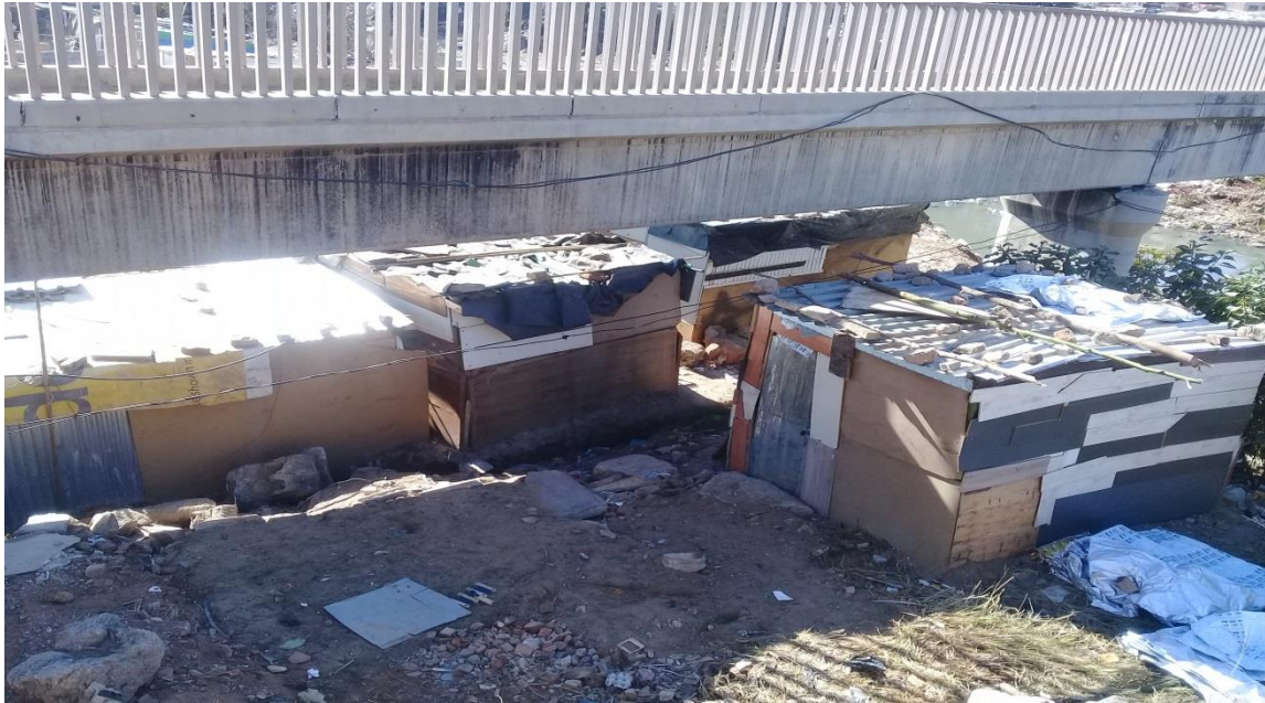
Figure 4.28: New shacks under the foot bridge at Jukskei River banks (03/07/2018).
