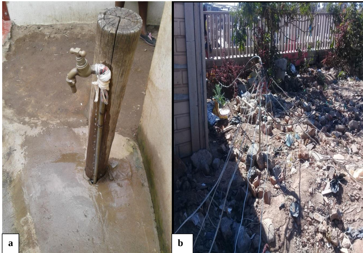
Figure 4.17: (a) Leaking community installed tap (01/03/2018) and (b) illegal electric connections (03/07/2018).
