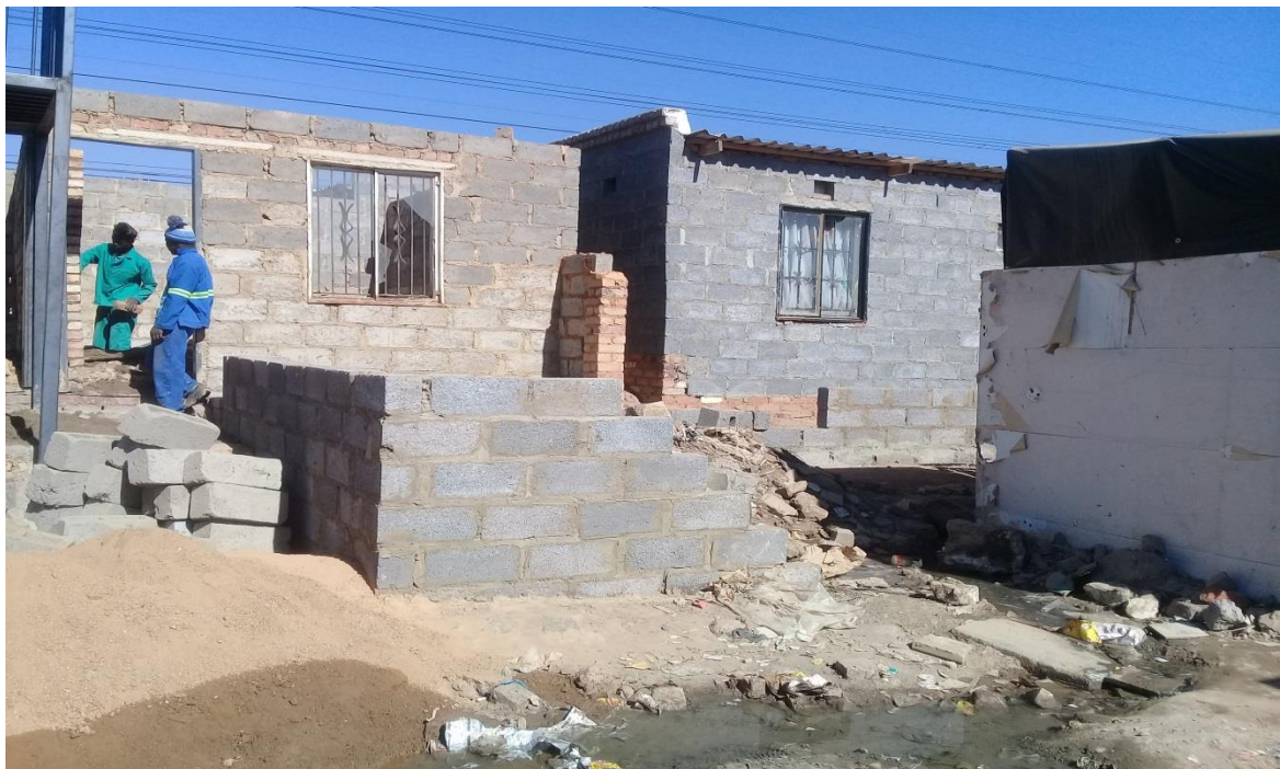
Figure 4.24: Houses built from new blocked bricks that were purchased in Setswetla (03/07/2018).
