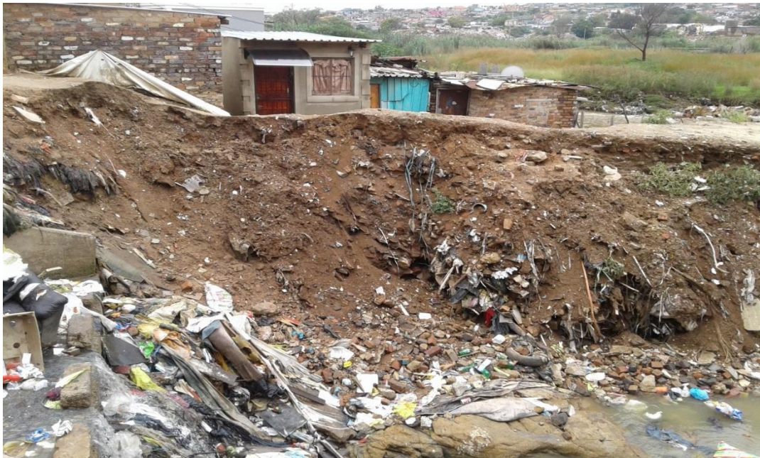
Figure 4.12: House built on layers of rubble and next to servitude of a sewerage pipe (23/03/2018).
