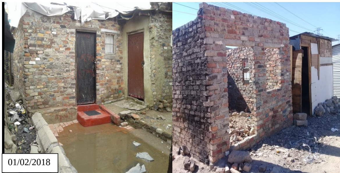
Figure 4.23: Houses built with rubble bricks (03/07/2018).
