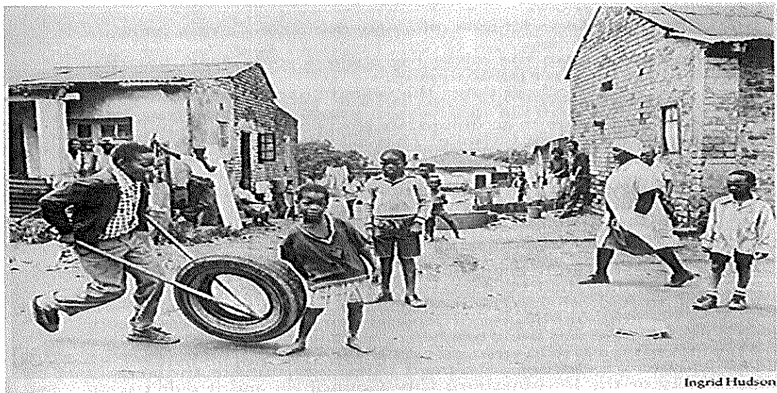
Figure 4.11: Reddish brick and corrugated iron housing (Alexsan Kopano Educational Trust, accessed 31/07/2017)
