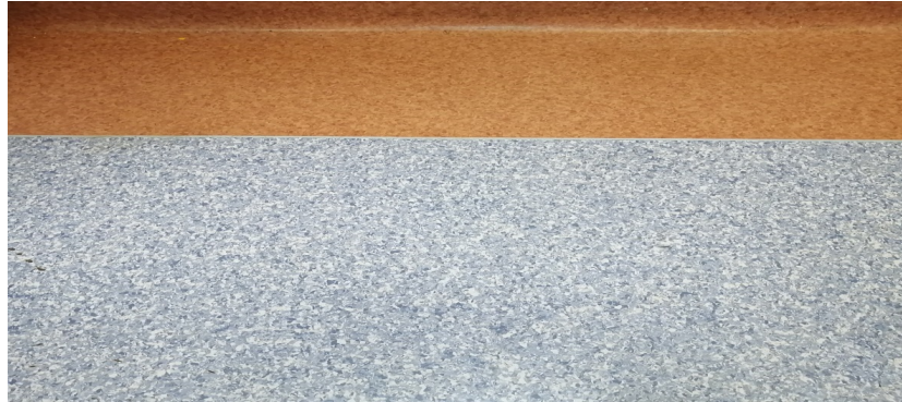
Figure 2.8: Picture showing the floor type in the DNM at CMJAH (with permission of the HOD). The floor is covered with a smooth and non-absorbent material.
