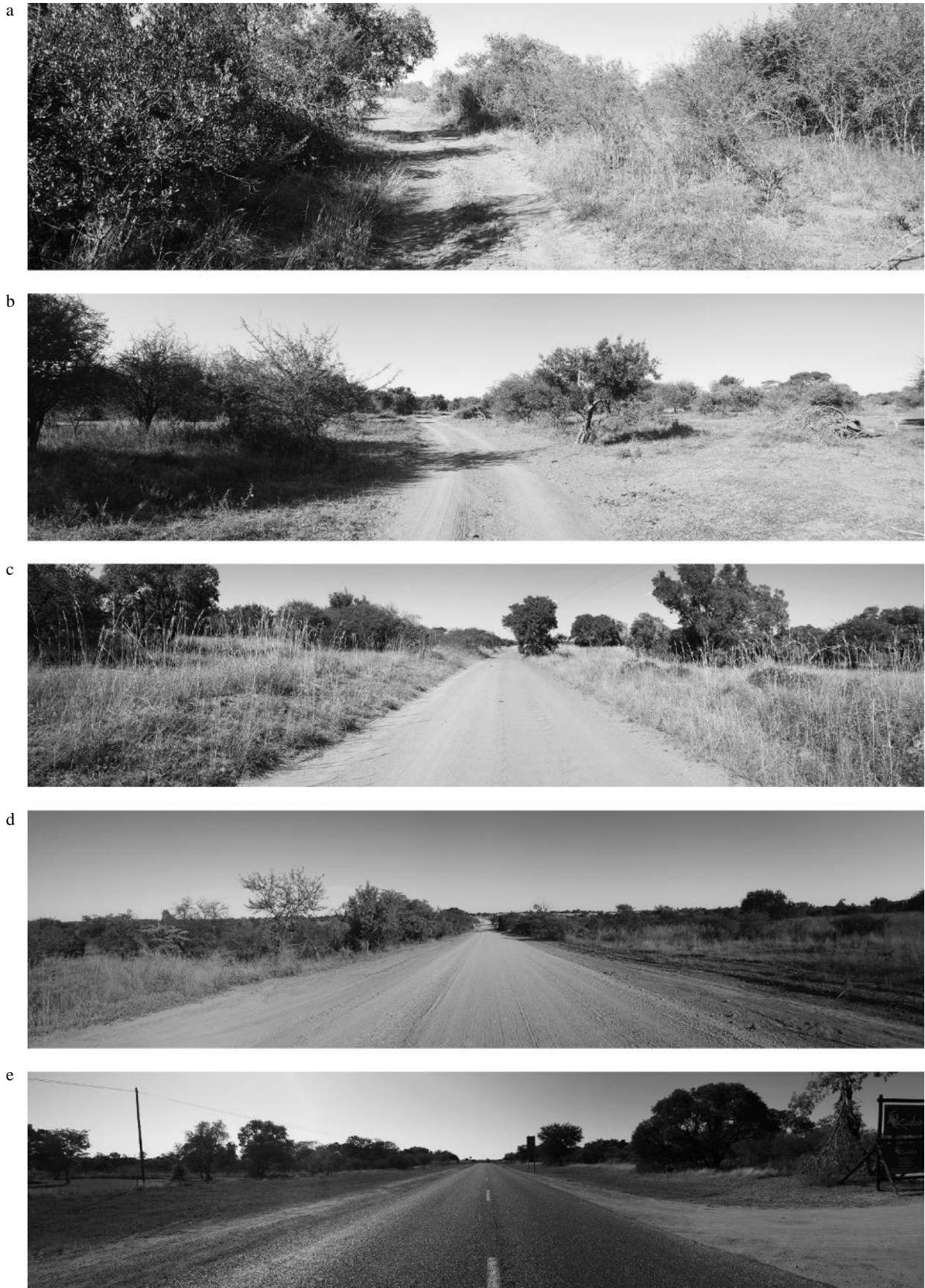
Figure 4. Examples of the various road classes identified in the Dinokeng Game Reserve. Letters 'a' to 'e' corresponds to the classes 1 to 5 respectively.
