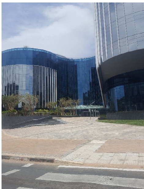
FIGURE 6: DISCOVERY BUILDING - VIEW FROM THE STREET
