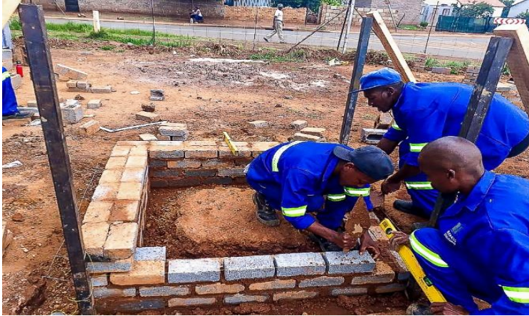
Figure 15: On-Site Bricklaying Skills Training in Lufhereng
