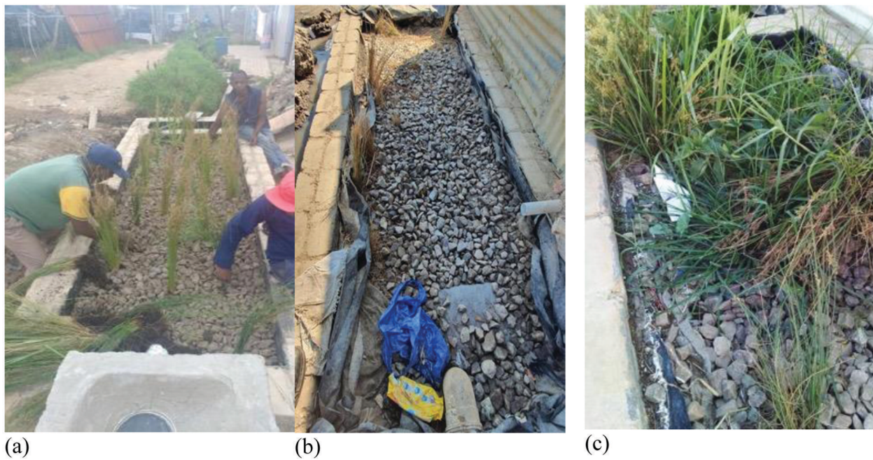
Figure 9. Interventions and their adaptation to environmental conditions shown as (a) the constructed wetland on final installation with nursery plants; (b) the constructed wetland after four months with all original plants dead; and (c) the constructed wetland after eight months.
