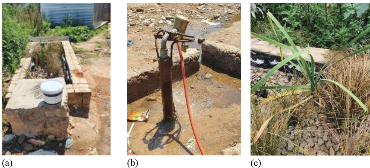
Figure 8. System adaptations where (a) a constructed wetland inlet being used as a table; (b) a broken communal tap because a community resident has made a direct connection to their own dwelling; and (c) a new plant species is growing in the constructed wetland that wasn't planted during construction.
