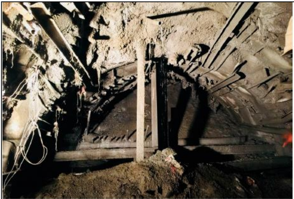
Figure 21 Temporary vertical struts for crown settlement control in DKHP (Diwakar et al. , 2022)
