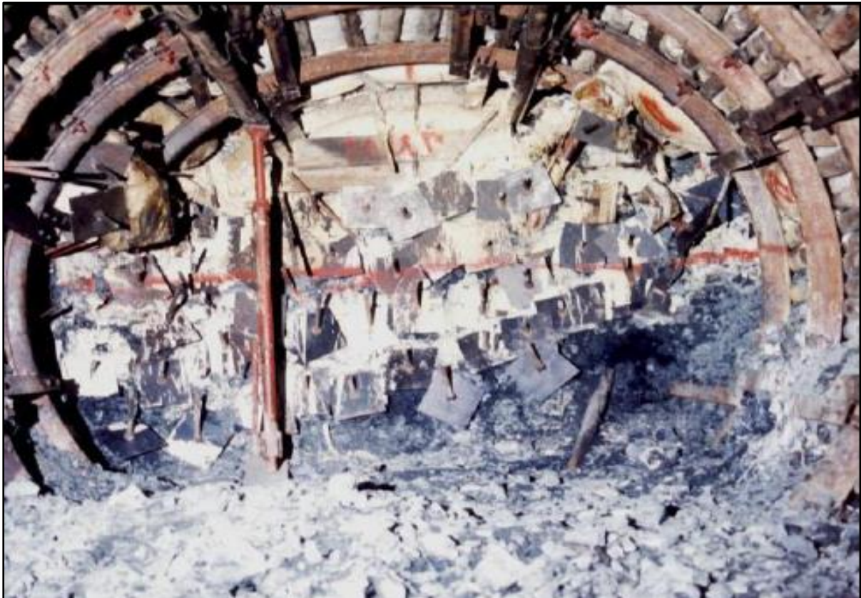
Figure 26: Ring sets with timber and void fill and consolidation bolts on the face (Oelofse & Judeel, 1999)
