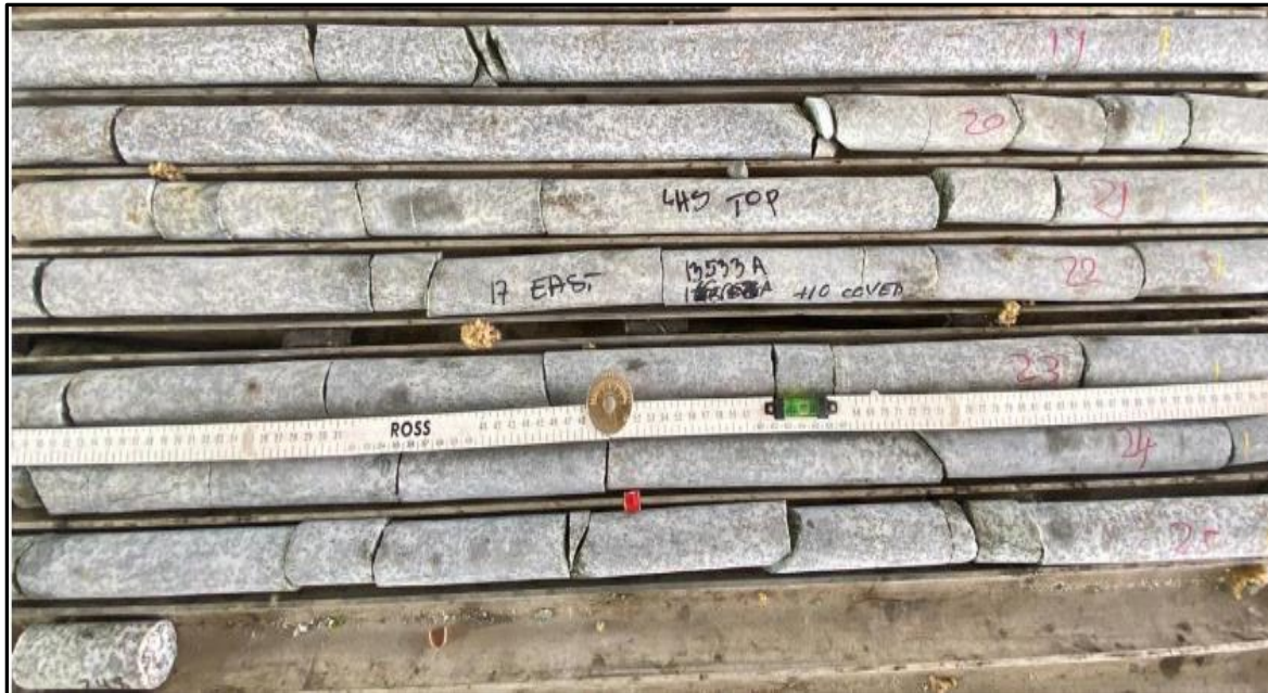
Figure 38: Borehole showing steep dipping joints recorded at Borehole HD 14072 m 19-25m Figure 39 reveals shallow dipping joints and partially altered joints. The core yielded low values of RQD due to closely spaced joints. The availability of water in this region significantly contributes to the decline in both the Q rating and MRMR.
