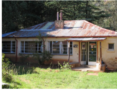
Figure 3: Building housing the Community Alcohol Rehabilitation Programme (CARP)
