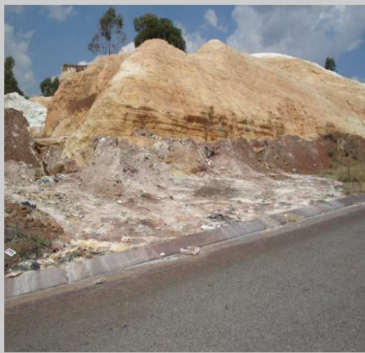
Position C facing east – shows eroded tailings leaving the TSF.
