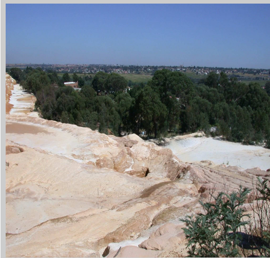
Position D facing west – shows eroded tailings leaving the TSF.
