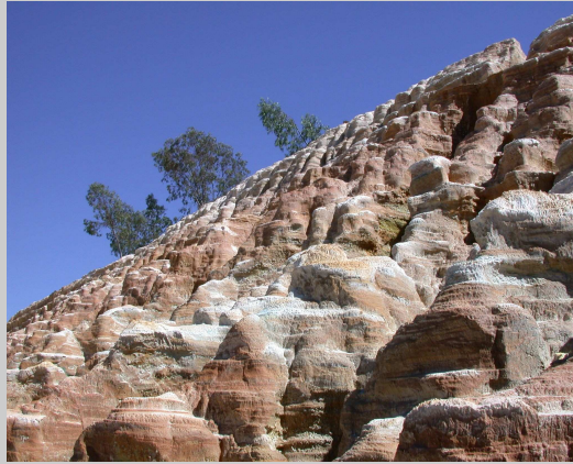
Position A facing south – Showing the impact of erosion on the unprotected slopes.
