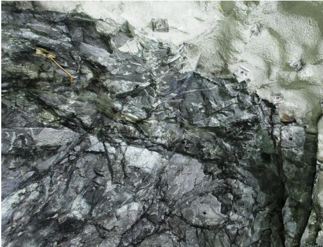
Figure 4-2: Shows Site a jointed rock mass (Masole, 2022).
