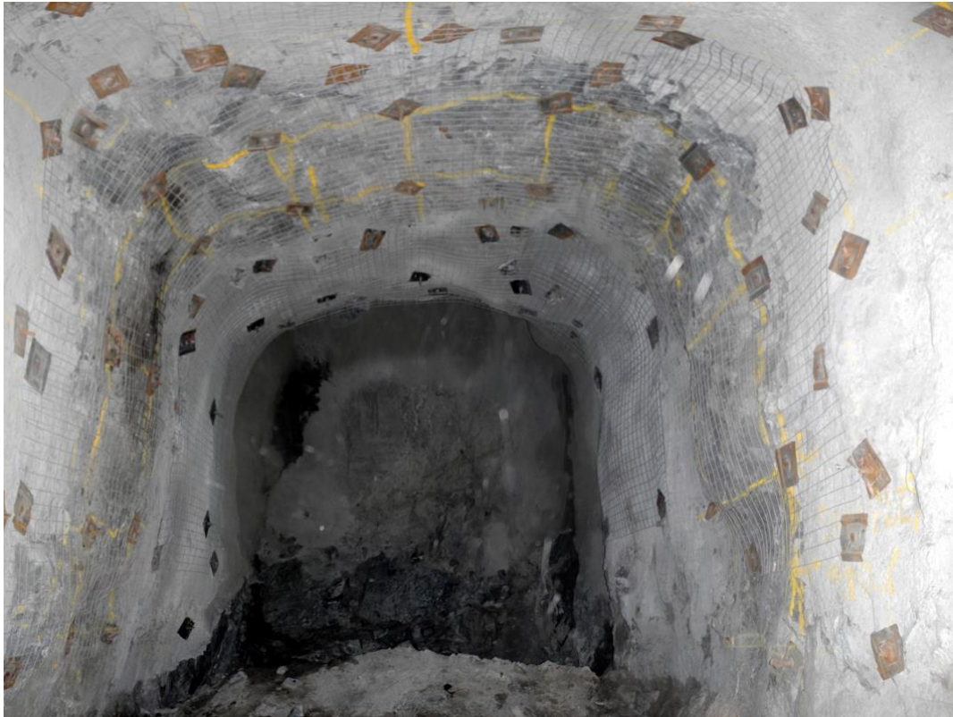
Figure 4-4: Illustrates an excavation with loose shotcrete held by mesh (Masole, 2022).
