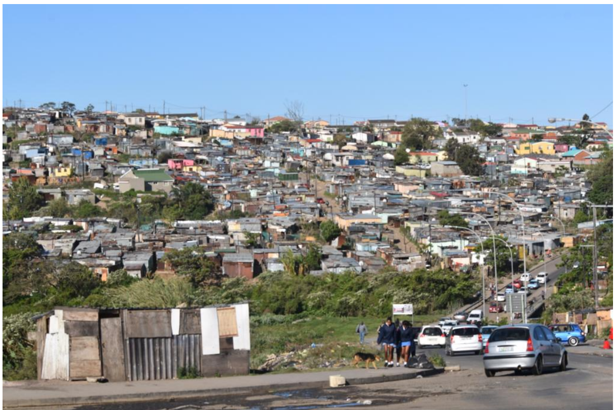
Image 25: A view of Duncan Village Proper from the Ford Traffic Circle on Douglas Smith Highway.
