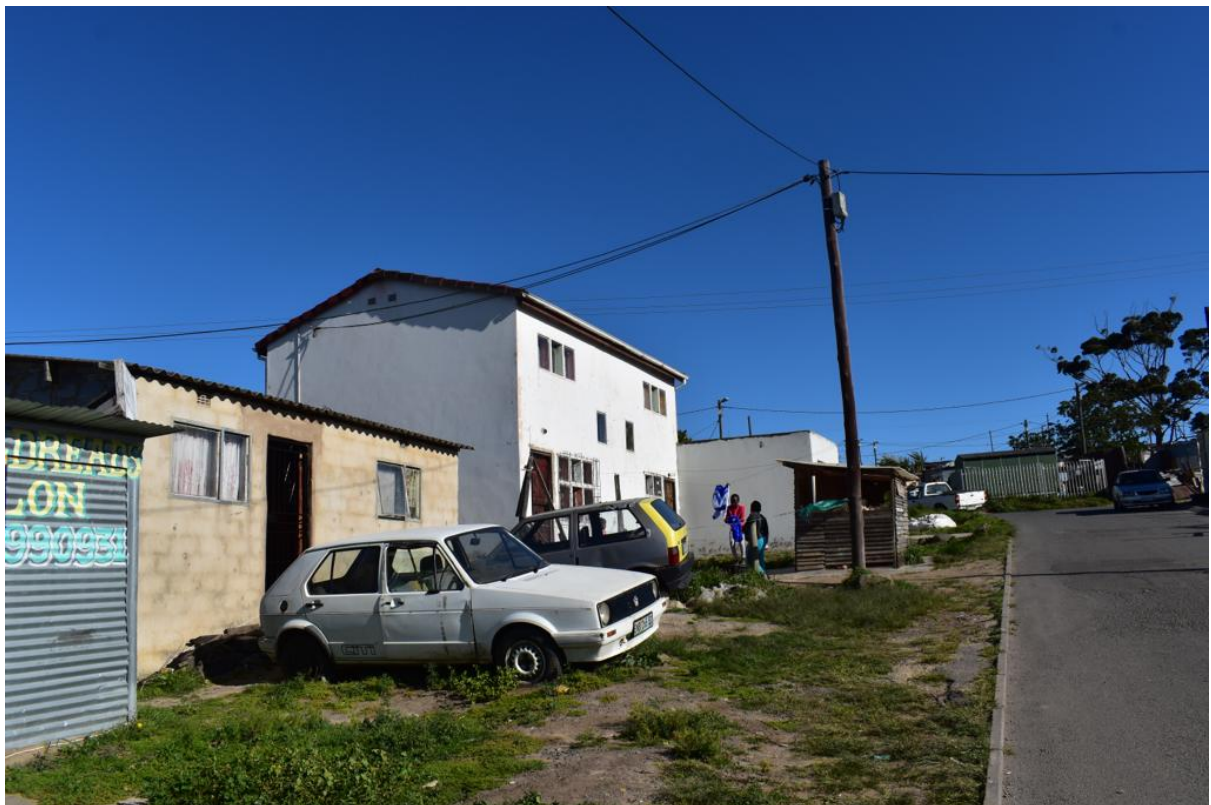
Image 21: The first pilot house for the Duncan Village Redevelopment Initiative (DVRI) project (see Chapter 1 ).
