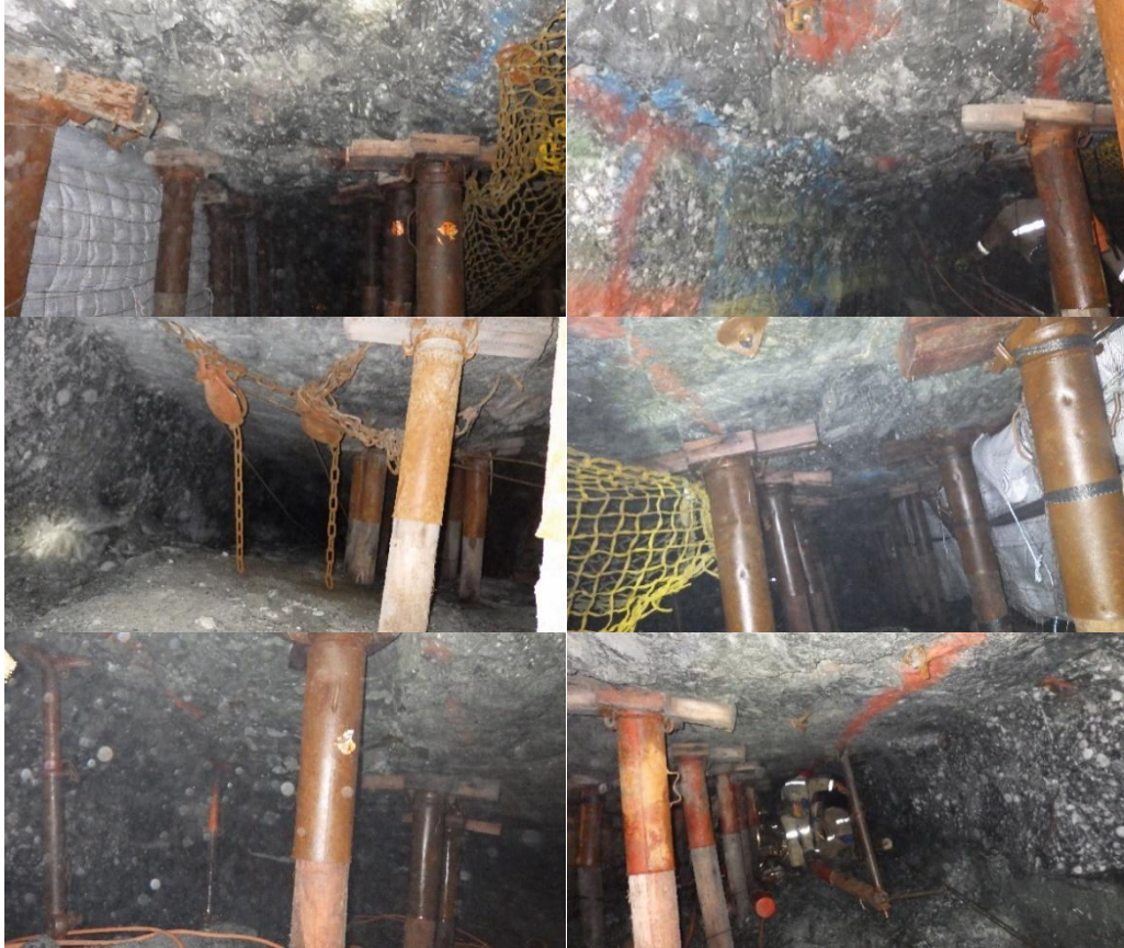
Figure 4.2: Photos from different stopes showing the generally smooth hangingwall conditions in the east mine stopes
