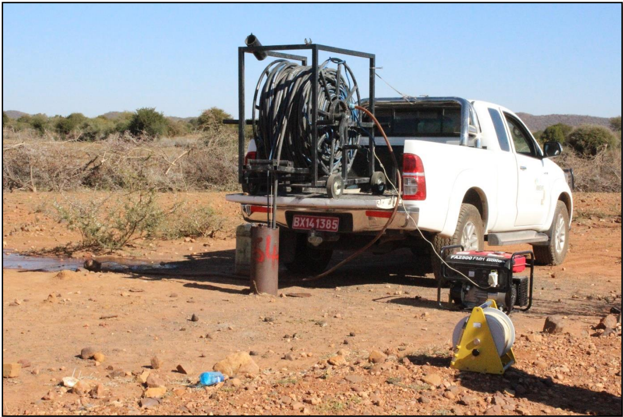
Figure 15. Well purging after uncapping the borehole.
