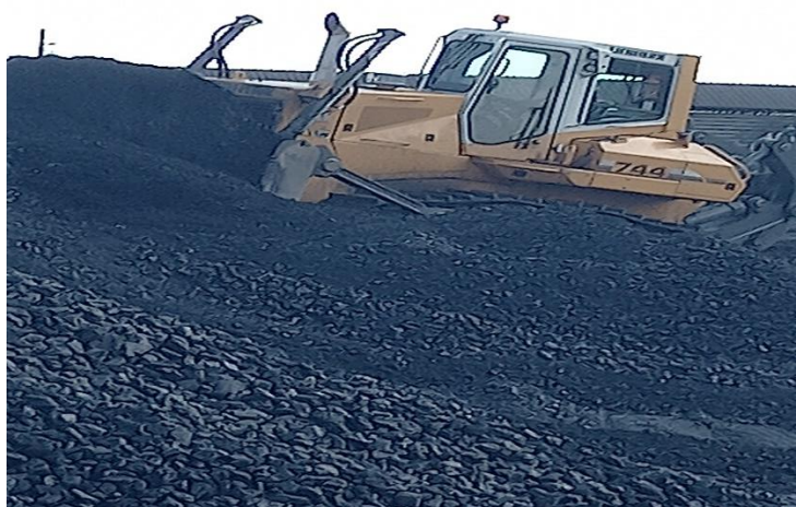
Figure 2: Typical Bull dozer working on coal stockpile.
