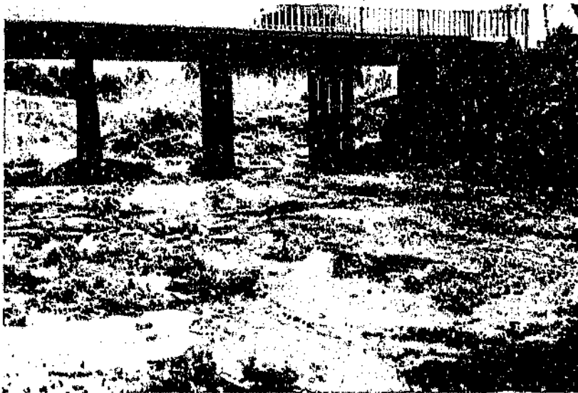
Monitoring point 2 (JUK2) - (Frankenwald/Marlboro Drive)
