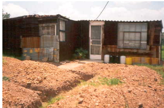
'PHP' Foundations in front of shack
