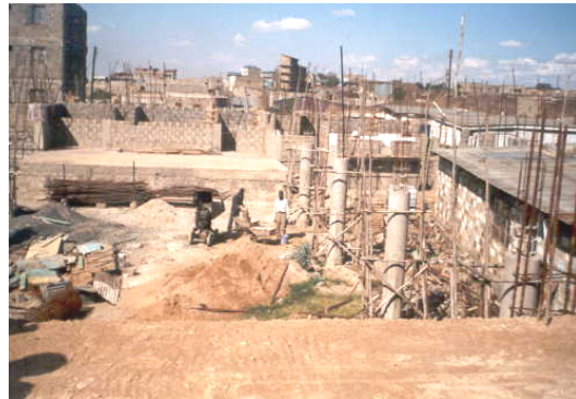
R.C. construction in Dandora
