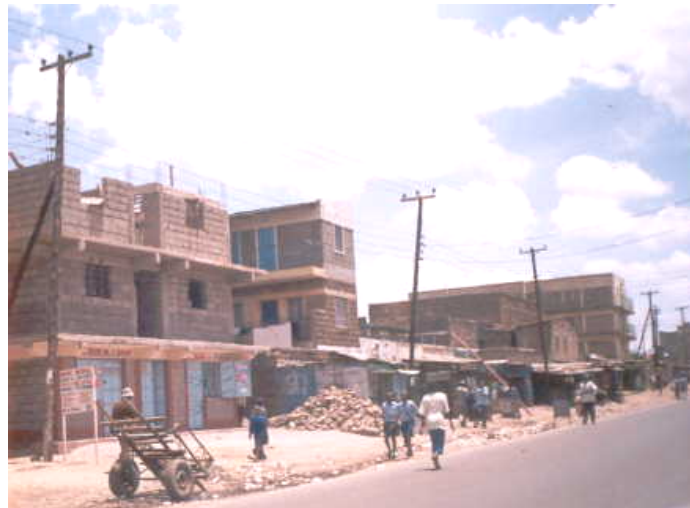
Incomplete construction in Dandora
