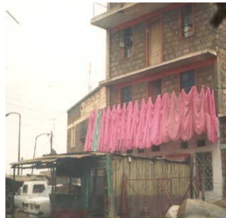
Shack in front of a tenement in Dandora
