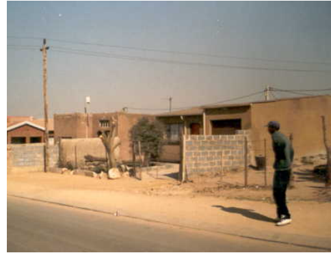
Consolidation on serviced sites
