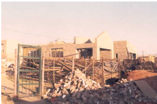
Material piling in Diepsloot
