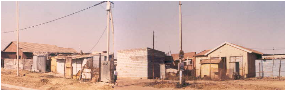
Consolidation and coexistence between formal and informal developments Ivory Park, Johannesburg
