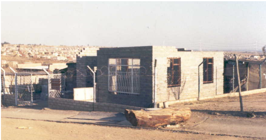
Typical construction in Diepsloot
