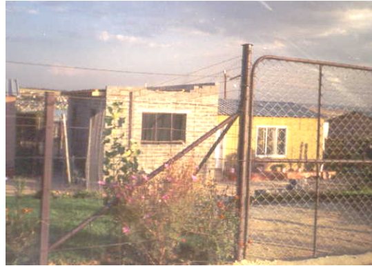
Consolidation of RDP house
