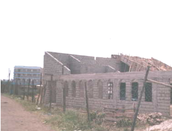
Construction in Dandora Dandora, Nairobi
