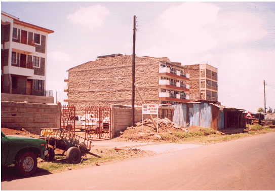
Construction on road reserves in Dandora
