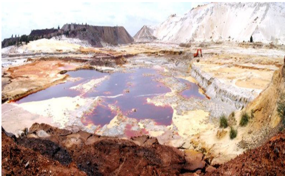
Plate 4.2 Unrehabilitated slime dam (Source: Leon Croukamp, CGS).
