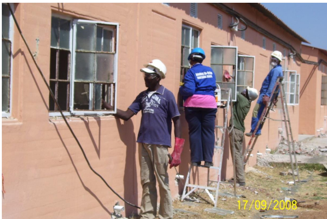
Photograph 4.12 Construction workers, including women, installing and cleaning windows
