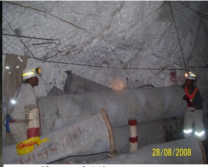
Photograph 4.10 Transport women carrying ventilation pipes from one section to another
