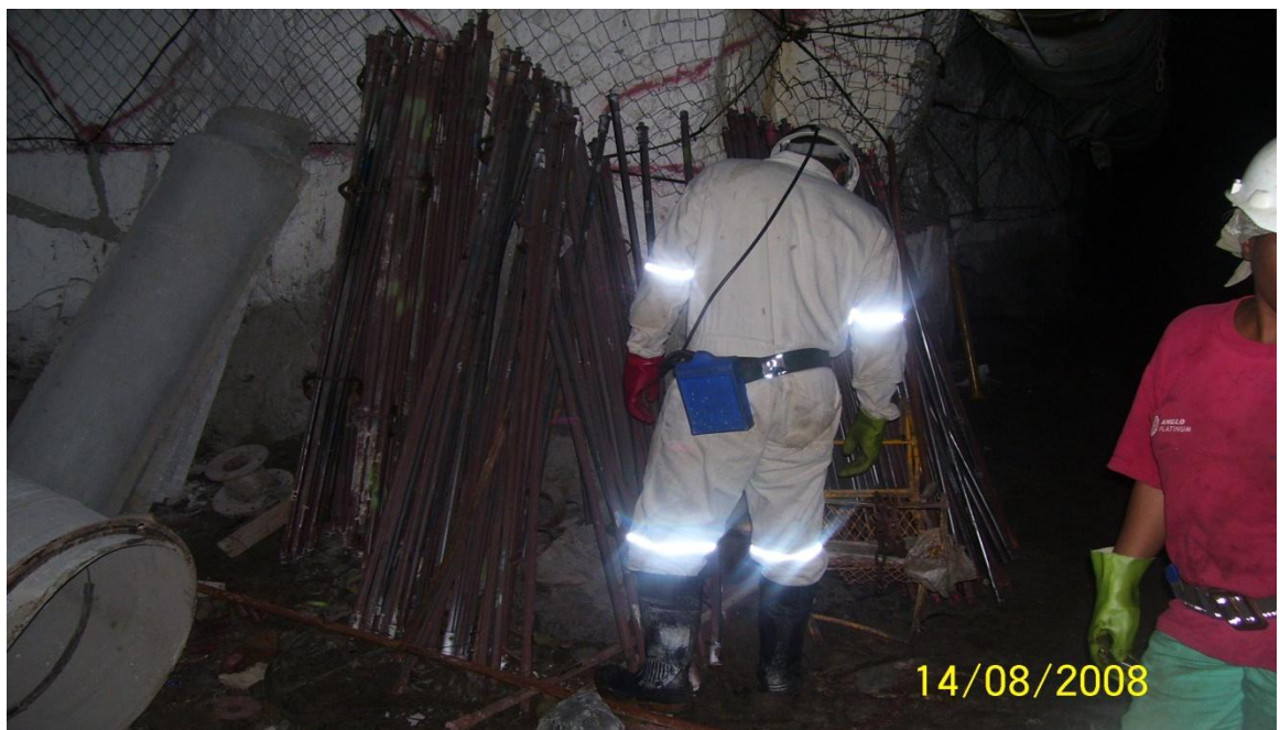
Photograph 4.17 Workers about to take roof bolts and pipes to their working stations
