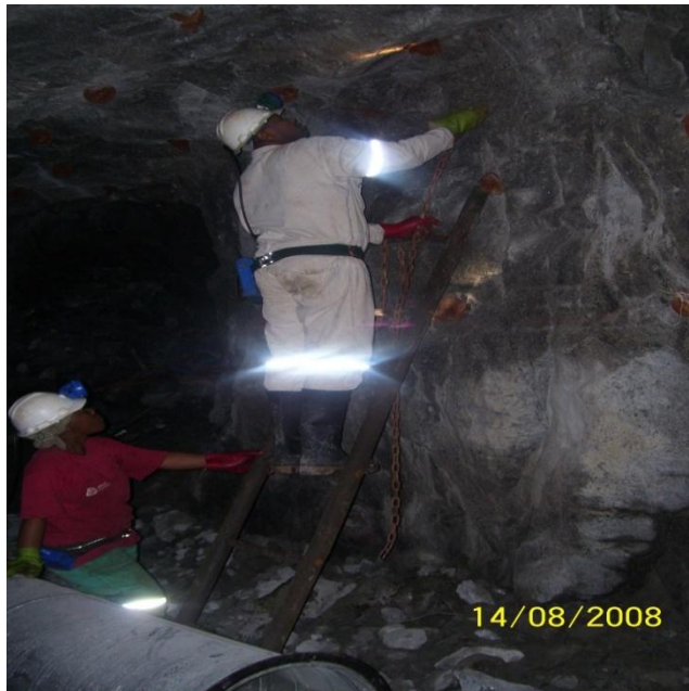
Photograph 4.8 A female worker assisting a male co-worker install a ventilation pipe
