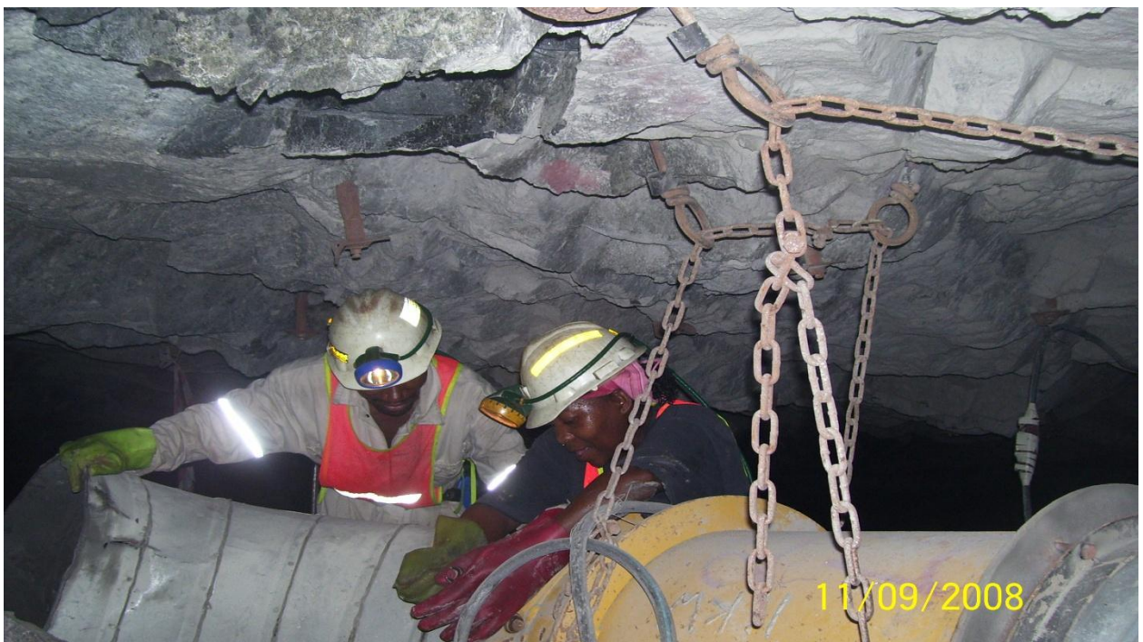
Picture xxx: A female worker extending a ventilation pipe
