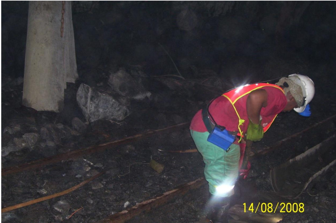
Picture: A female worker cleaning the drain and installing a railway line
