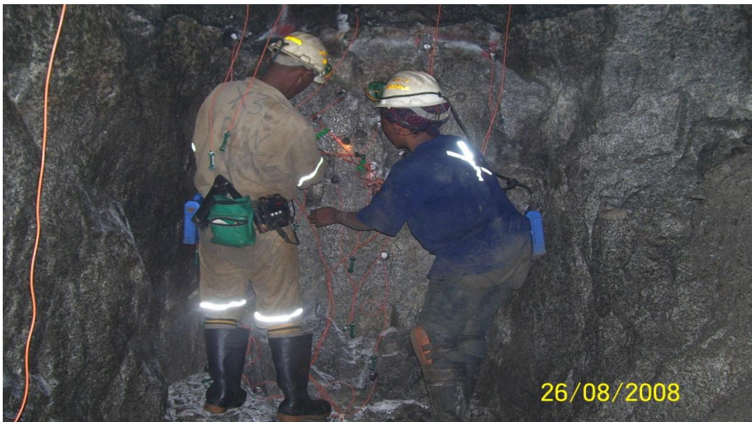
Picture: A female worker assisting a miner connect blasting cables
