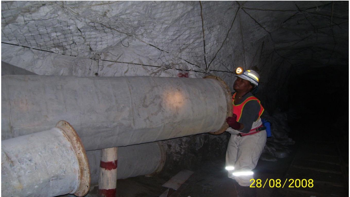
Picture: A female workers installing a ventilation pipe
