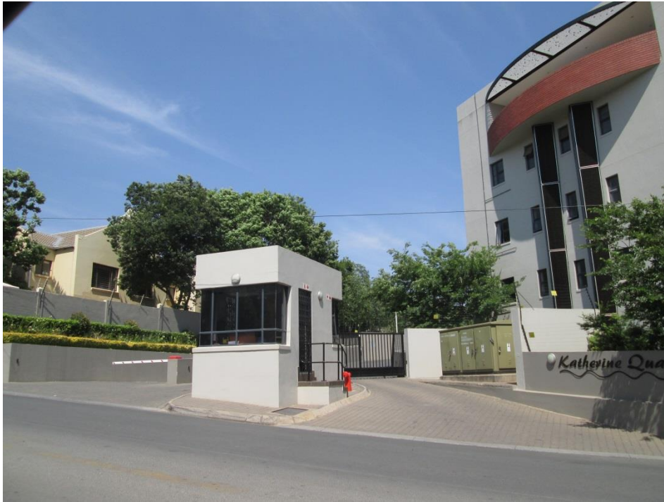
Figure 2: Apartment Complex in Sandton (Security features), (Mngaza, 2015)
