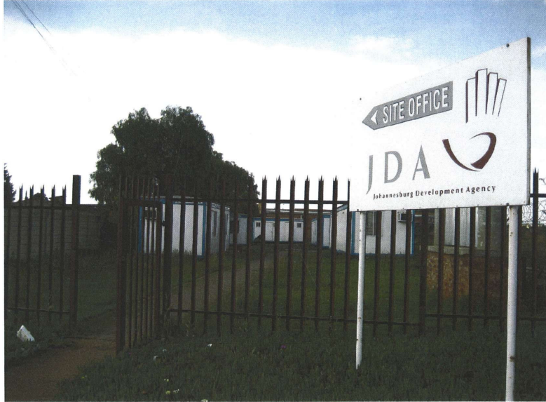
Abandoned JDA site office
