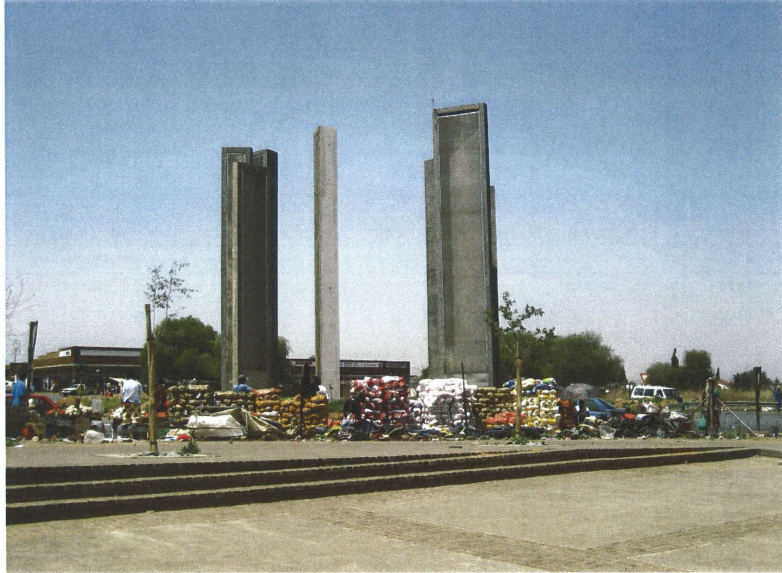
Concrete bollards at the traffic circle on Union Road with traders. . .
