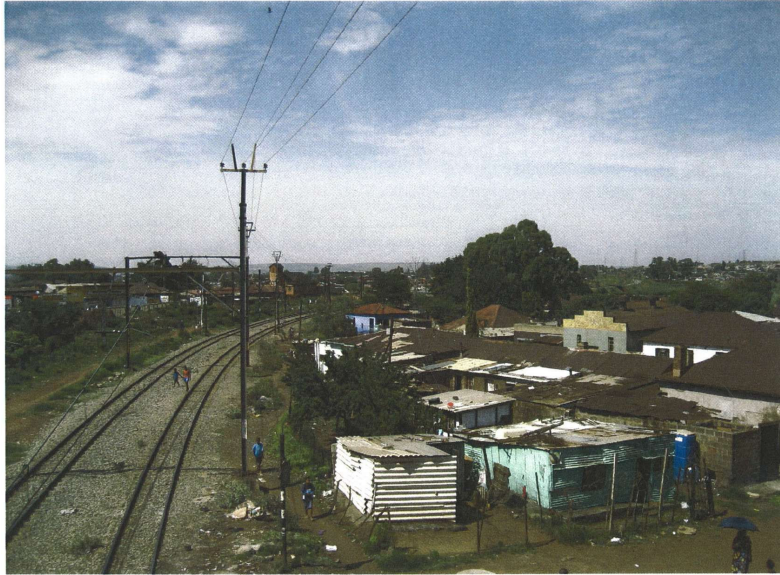
View from pedestrian bridge. Intersection of Union and Station Roads.
