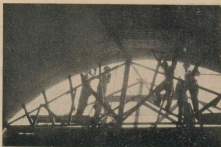
Photo No. 2. Temporary truss supporting rings during fixing.
