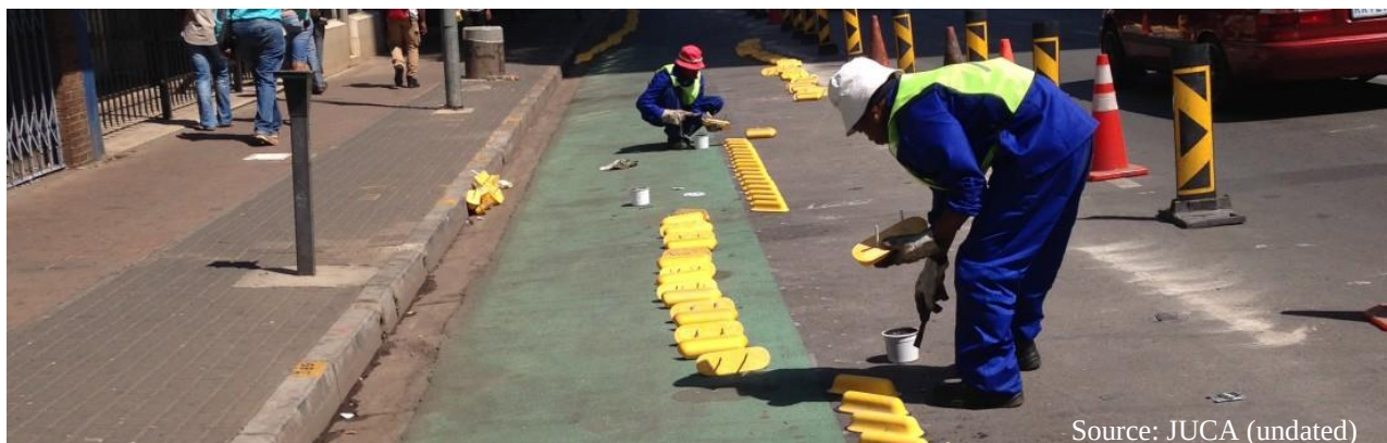
Figure 13: Construction of the bicycle lanes in Braamfontein
