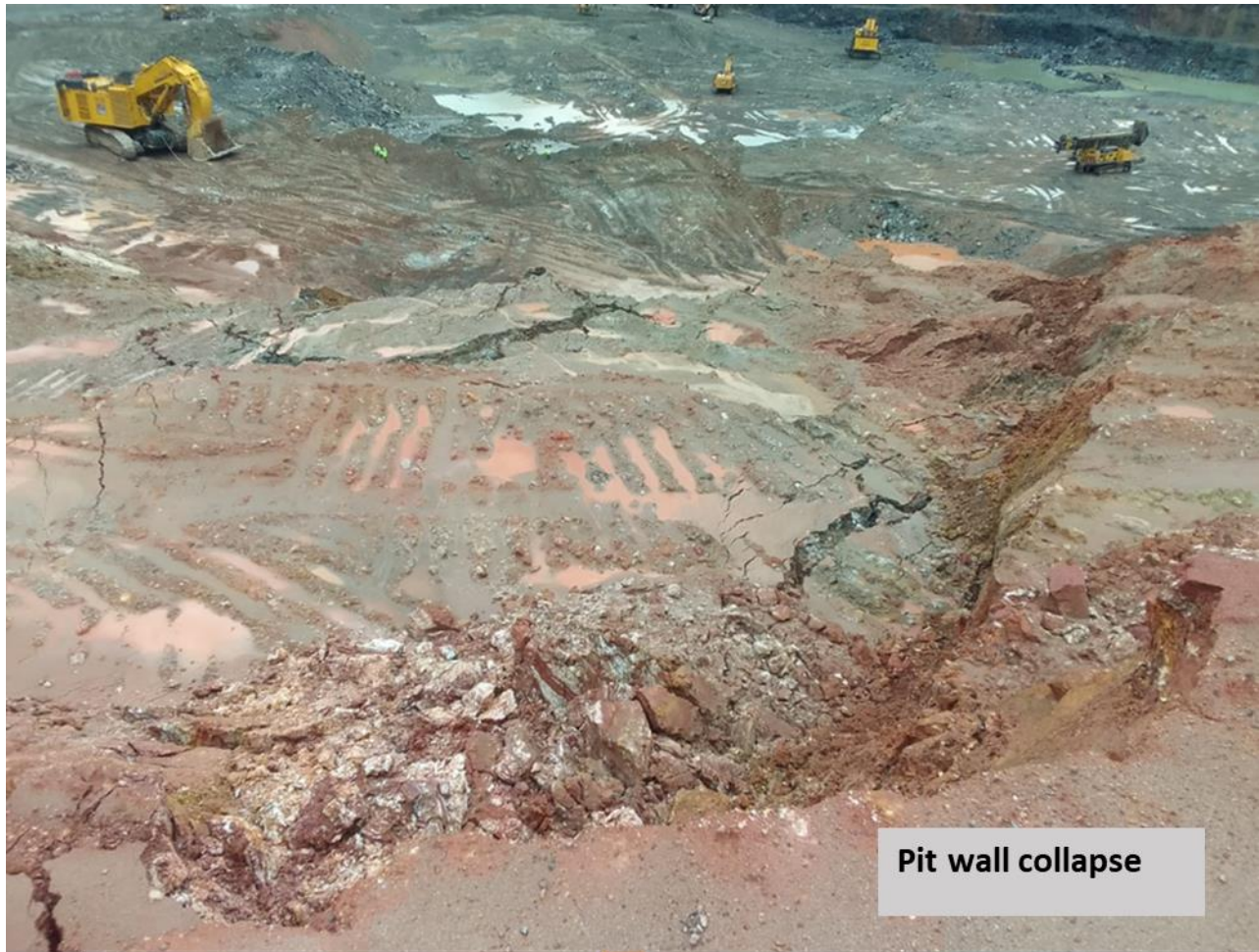
Figure 1.2 Example of pit wall failure in the weak saprolite zone along a fault plane at Lumwana Mine. Note the saturated ground floor below the failure. (Source: Lumwana Geotechnical Engineering Department).
