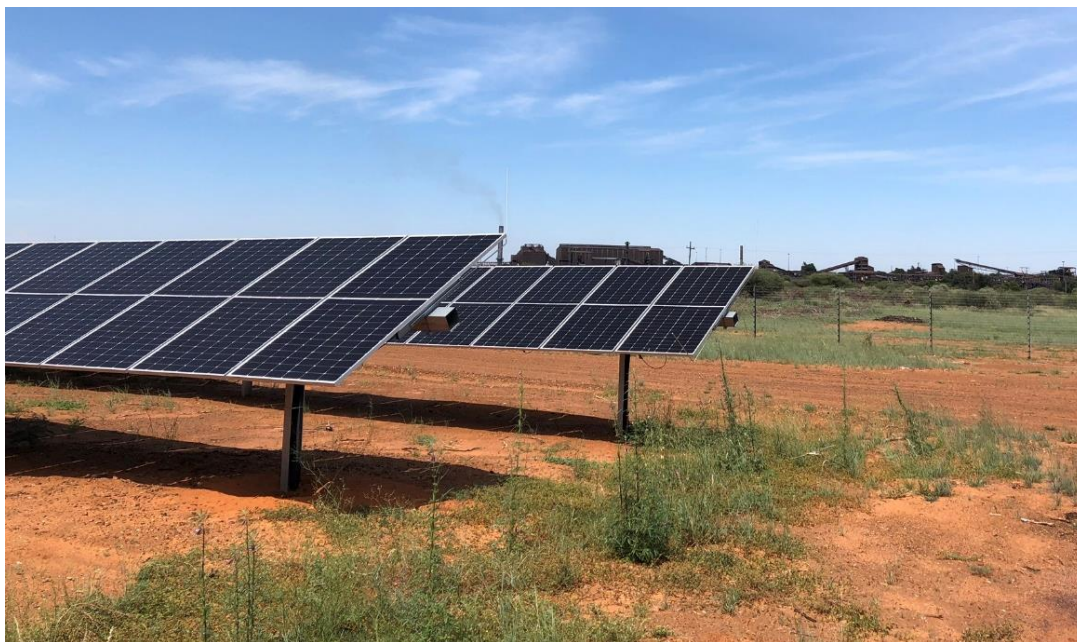
Figure 4: A solar power plant opposite a manganese mine near Kathu, Northern Cape.
