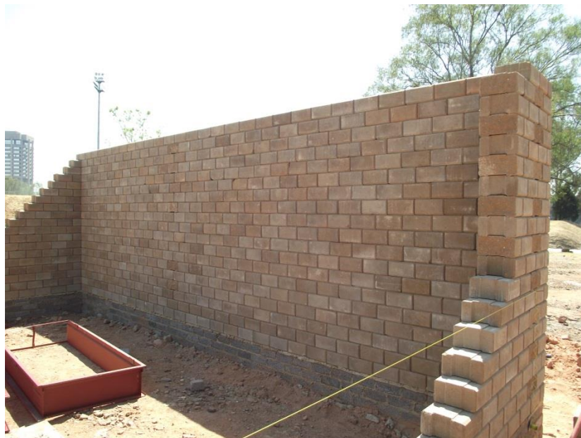
Figure 8-11: A completed dry-stack wall
