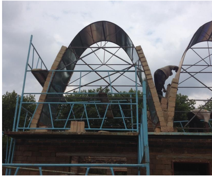
Figure 8-34: Constructing on each side to prevent swaying of the formwork under the weight of the vault
