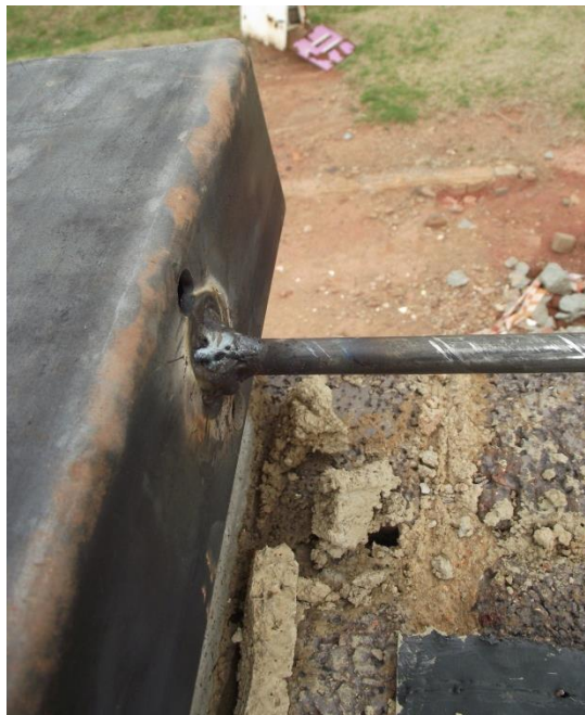
Figure 8-24: The steel ties are welded to the tubes at the ends of the structure
