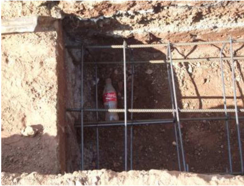
Figure 8-3: Holes are drilled into the raft foundation so that the edges of the steel cages can be connected into the raft
