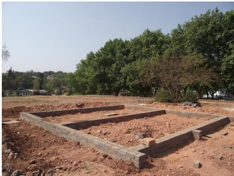
Figure 8-7: The cement bricks are built to 300mm before the dry-stack layers begin
