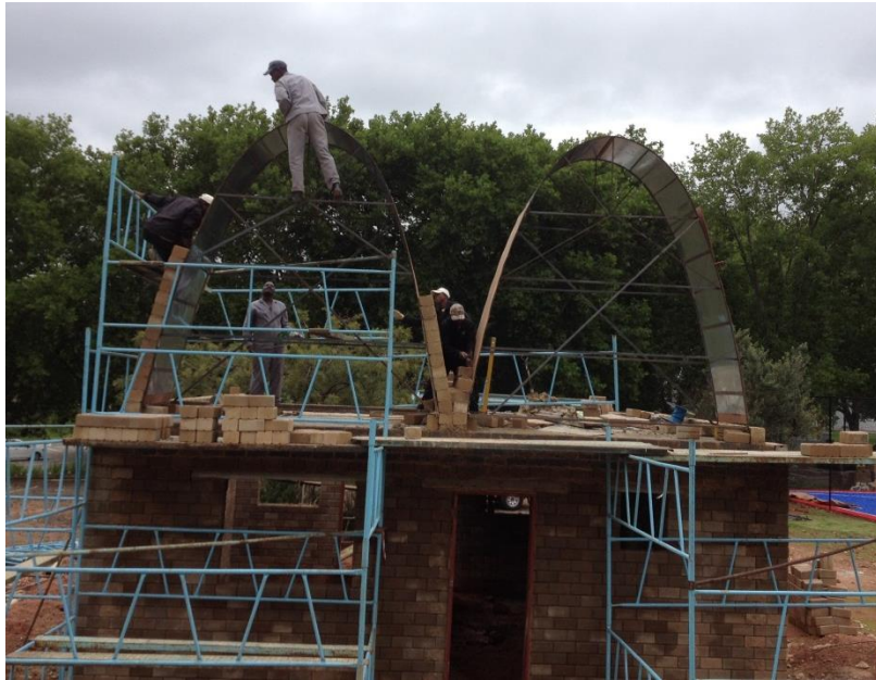
Figure 8-31: The start of the construction of the vaults
