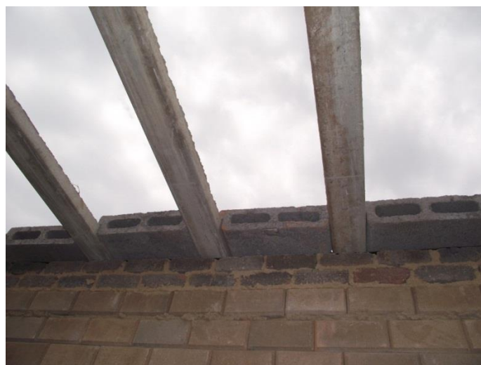
Figure 8-19: Placing the blocks between the ribs
