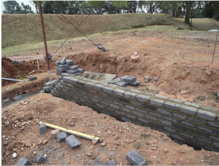
Figure 8-6: Cement bricks are used to construct the base of the wall to 300mm above ground level
