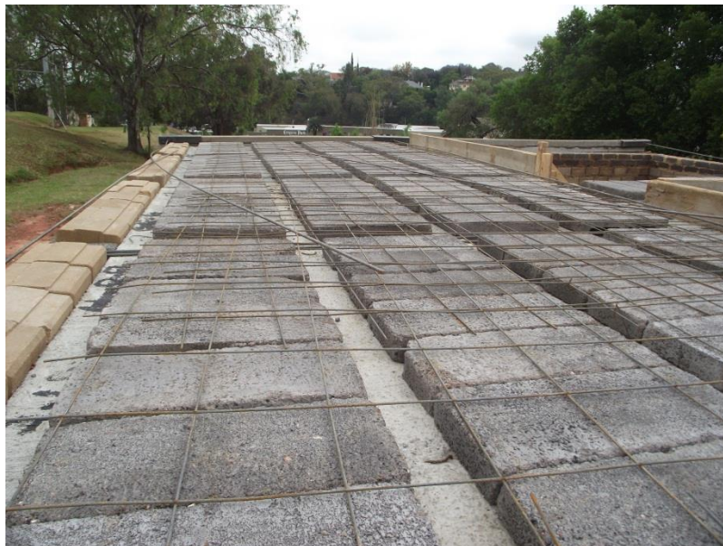
Figure 8-21: Steel mesh and reinforcing is positioned on top of the slab
