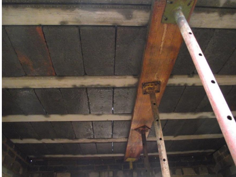
Figure 8-20: Props are set up under the slab to support it until concrete is poured
