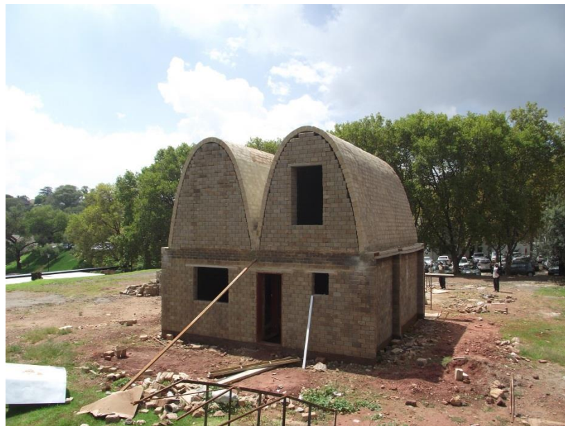
Figure 8-46: Completion of the top floor walls and thus the superstructure
