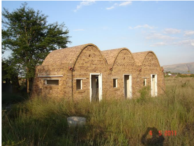
Figure 2-9: The vaulted roof in Bapong Township was constructed with a sliding formwork
