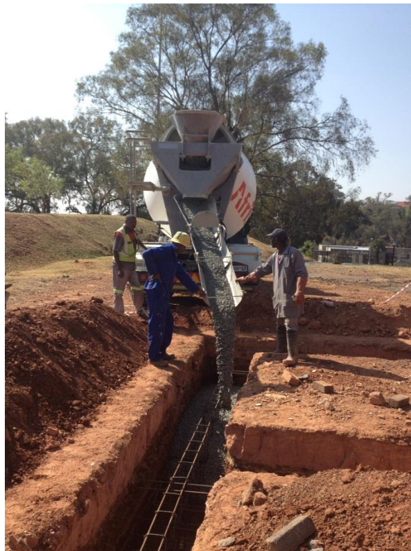
Figure 8-4: Readymix Concrete is poured into the foundation
