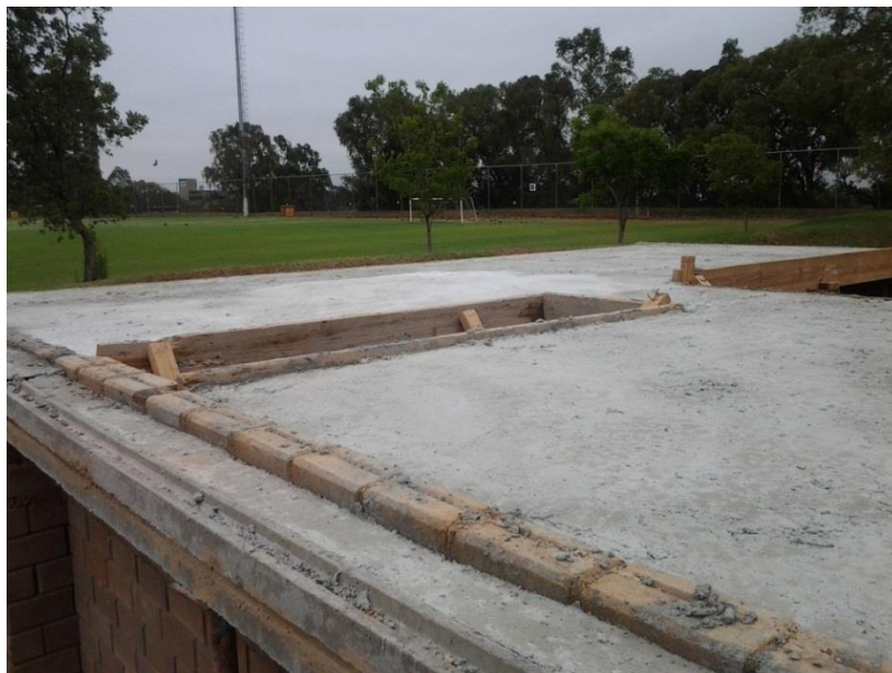
Figure 8-23: The final concrete pour; the slab is no complete and left to cure
