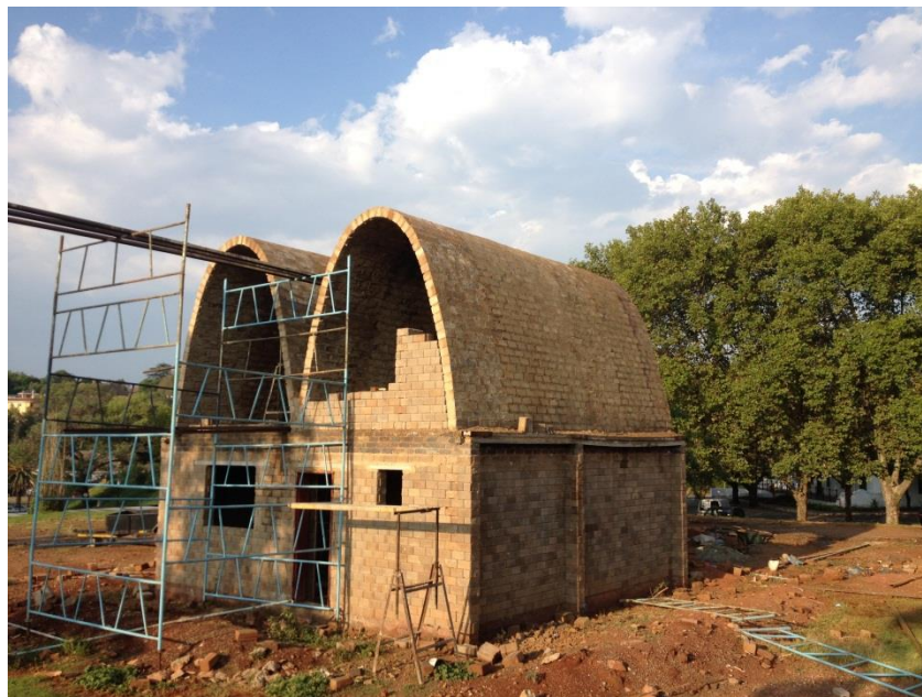
Figure 8-44: The completed catenary roof
