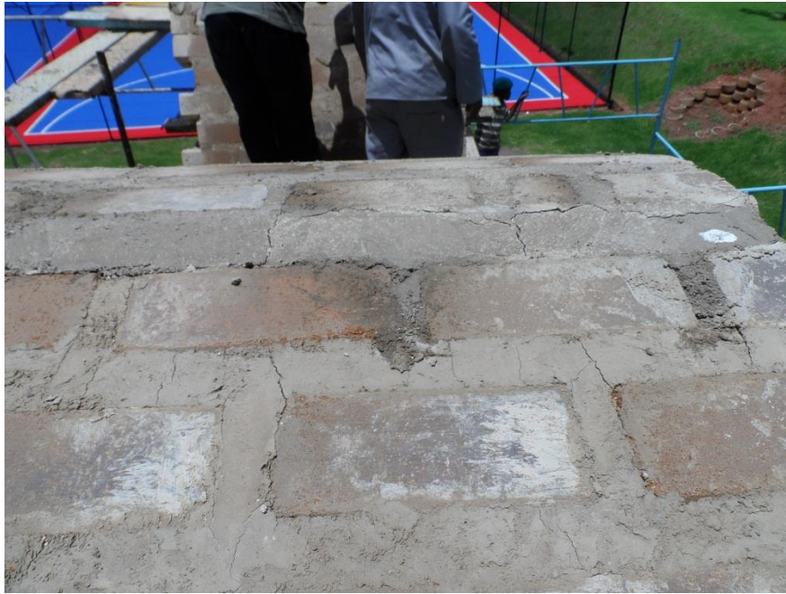
Figure 8-35: Cracking occurred along the apex as the vault is restrained from contracting naturally Once the first layer was complete, the formwork was shifted, repositioned and construction could continue (Figure 8-36 to 8-37). This was repeated until the entire structure was completed (Figure).
