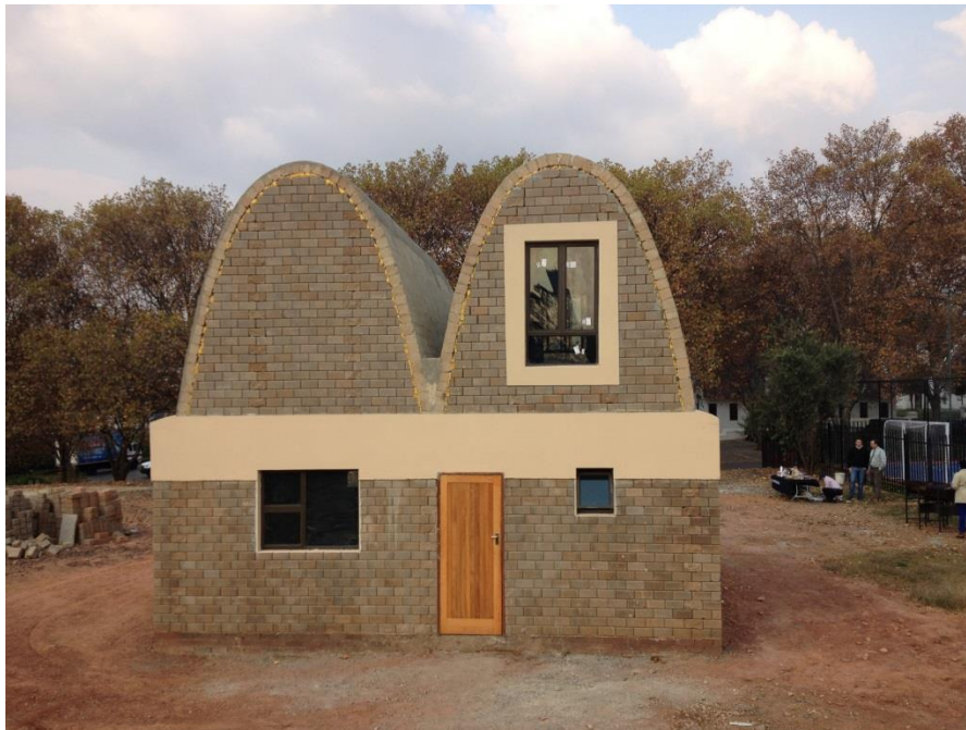
Figure 8-53: The completion of the painting concludes the construction of the structure
