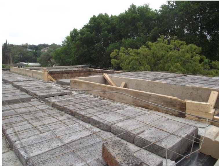
Figure 8-22: Wood shuttering is used around the openings
