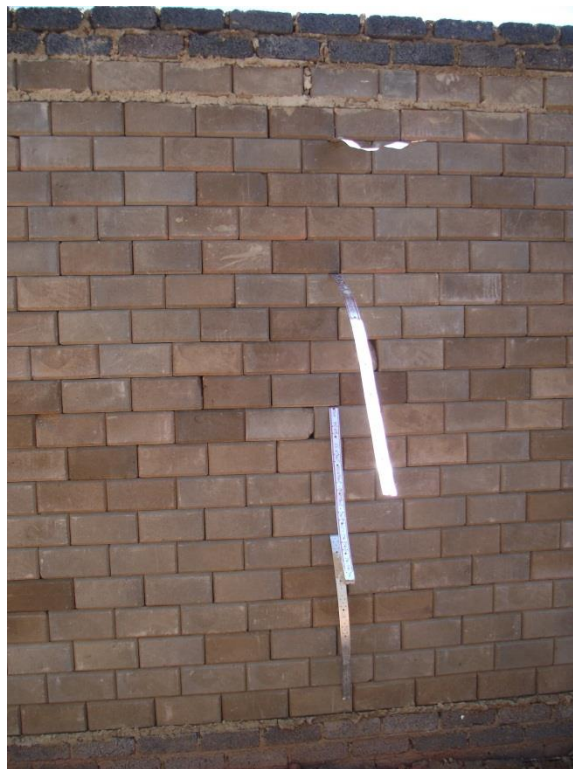
Figure 8-15: Ties are placed in the wall to connect the exterior and interior walls at a later stage
