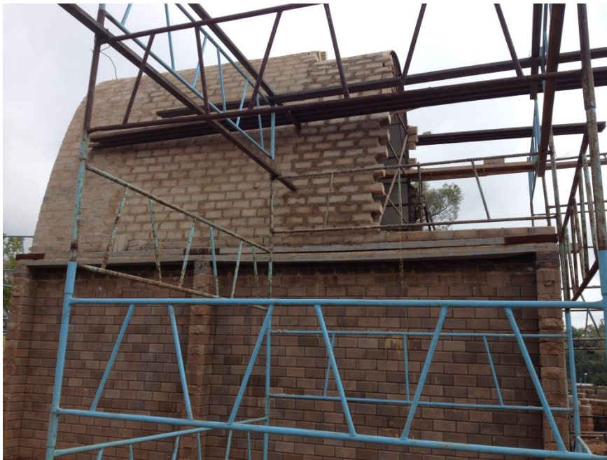
Figure 8-40: The construction of the vaults continues
