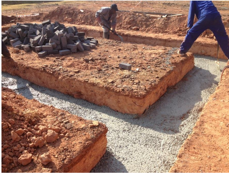
Figure 8-5: A 10mm layer is positioned over the entire foundation to bind the old and new concrete properly
