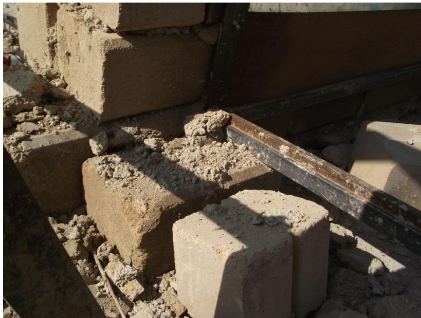
Figure 8-29: The formwork is propped up onto bricks which can easily be pulled out
