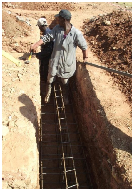
Figure 8-2: The steel sections are assembled into the inverted T shape and dropped into the foundations
