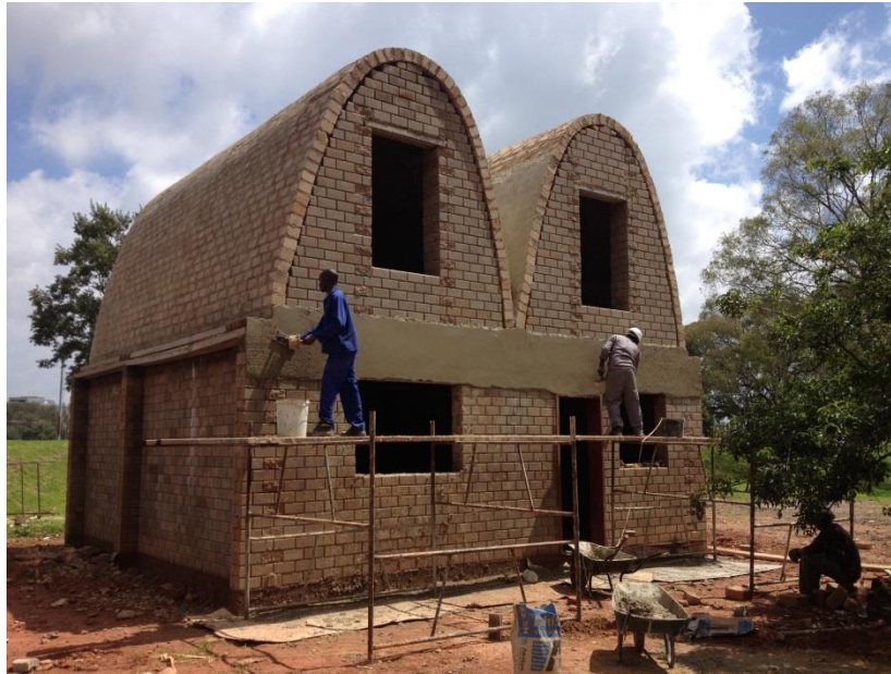
Figure 8-50: Plastering of the structure
