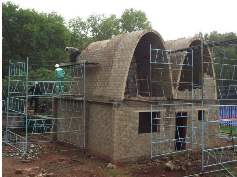
Figure 8-42: The second vault nearing completion
