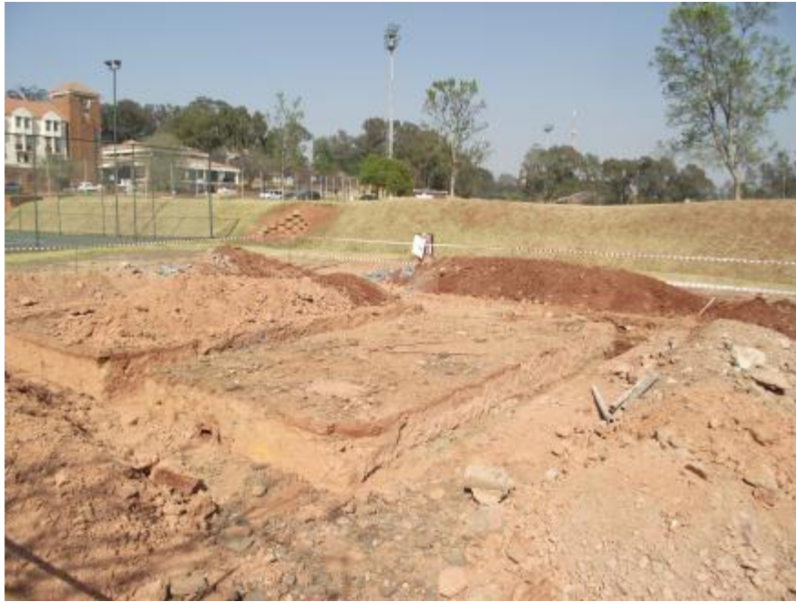
Figure 8-1: The foundation is measured and set up using builder's line before it is dug to the required depth
