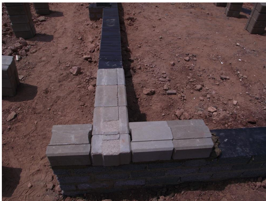
Figure 8-8: A layer of DPC is placed between the cement bricks and earth blocks
