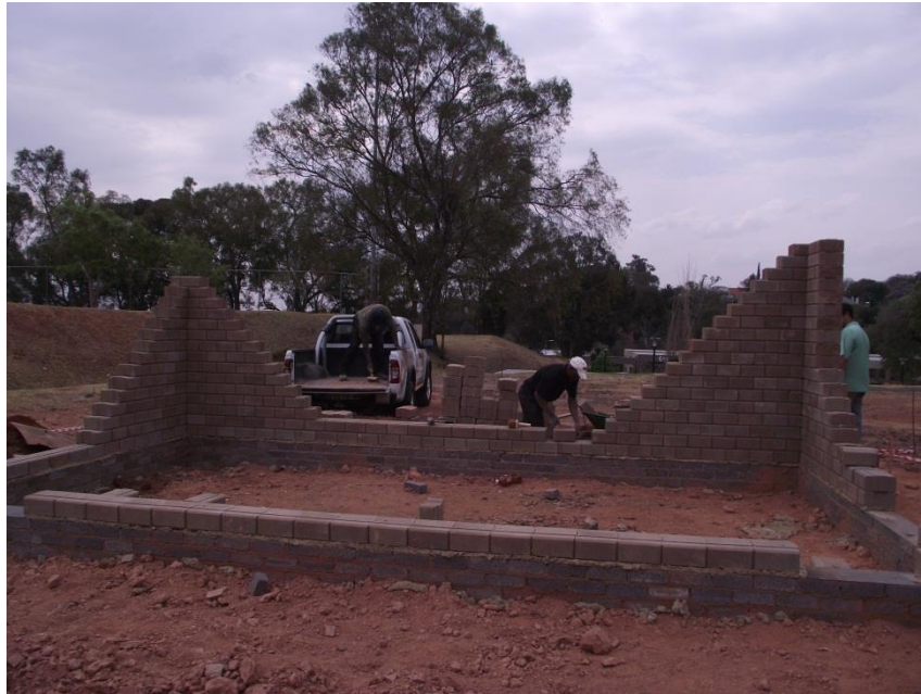
Figure 8-10: Construction of the walls is done from the corners-inwards
