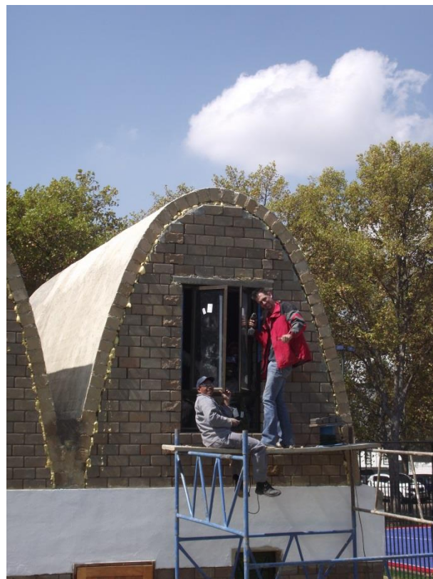
Figure 8-51: The installation of the windows
