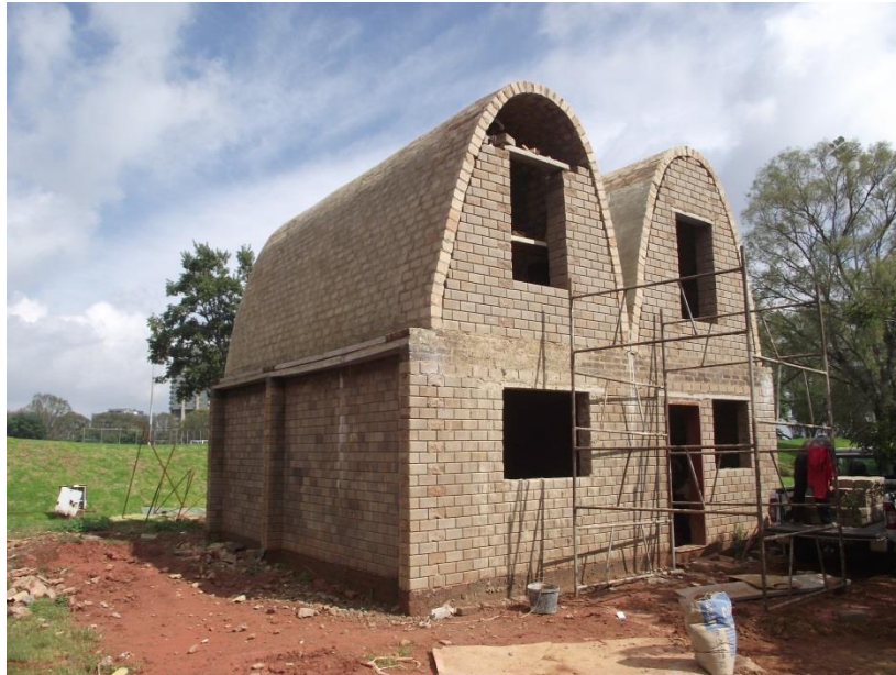
Figure 8-45: The construction of the top floor walls
