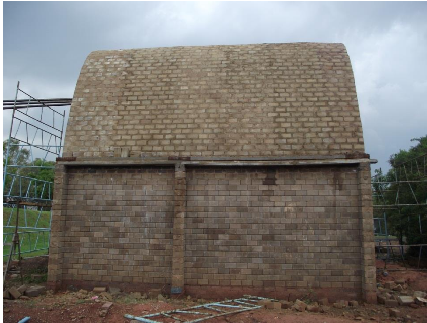
Figure 8-43: The completed vaulted roof
