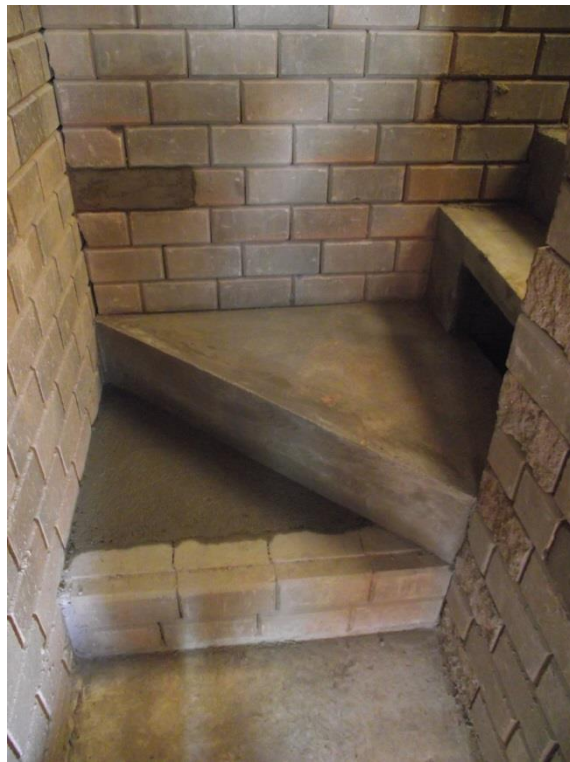
Figure 8-49: Construction of the staircase using lintels, blocks and mortar
