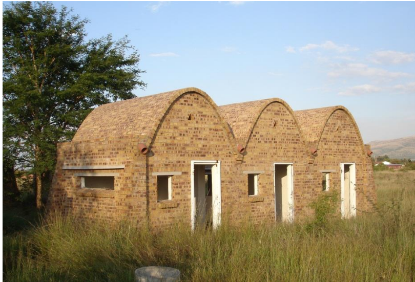
Figure 6-3: The abandoned structures are in impeccable condition even with no maintenance
