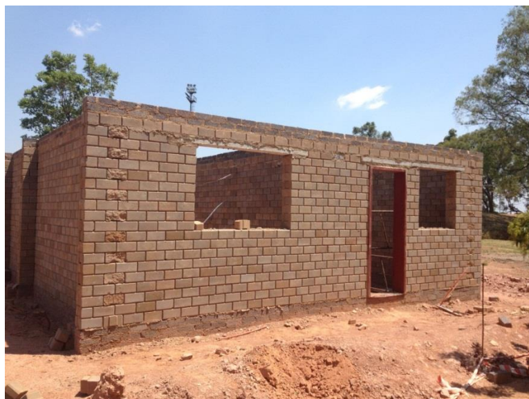
Figure 8-17: The completed first level, where the last two layers of bricks are cement bricks
