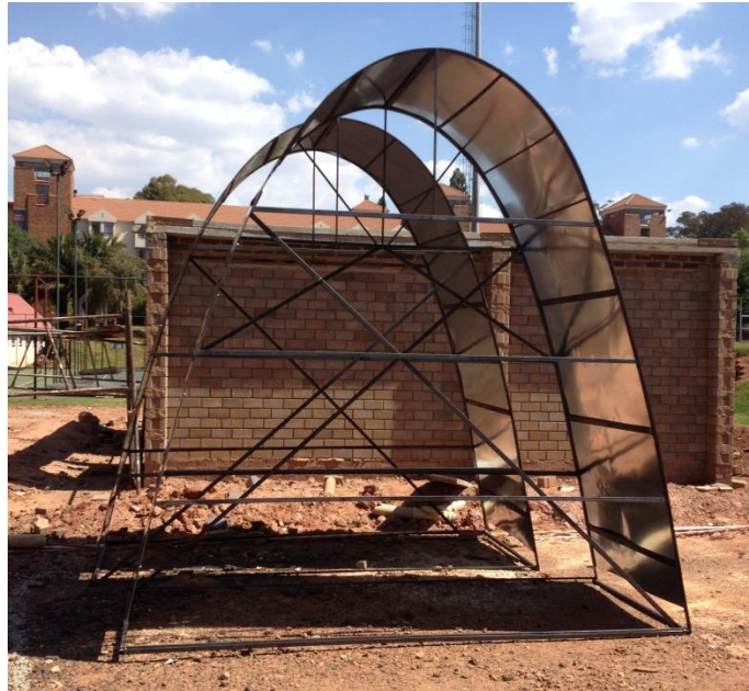
Figure 8-28: The two formworks at site, ready to be lifted and for construction to commence
