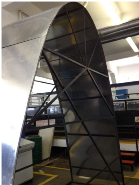
Figure 8-27: The steel formworks used to construct the vaults
