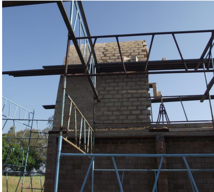
Figure 8-39: Construction of the second section is completed, the formwork is dropped and shifted and construction continues
