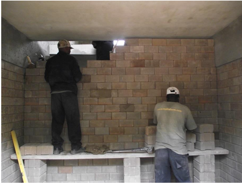
Figure 8-48: The construction of the internal walls
