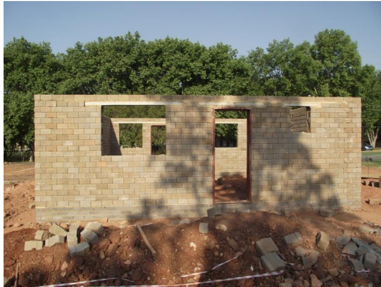
Figure 8-16: The completed walls with the last layer of dry-stack mortared in to lock the walls
