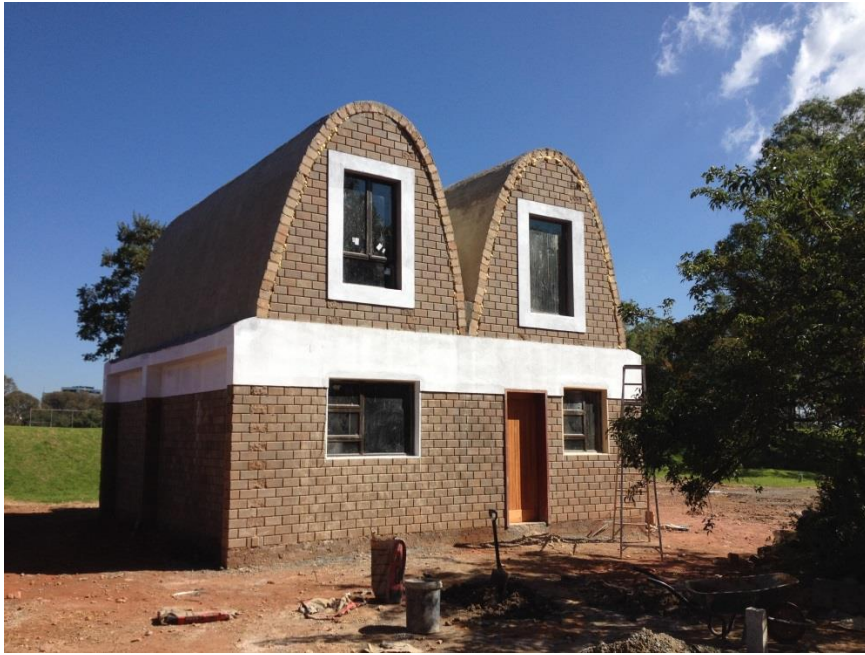
Figure 8-52: The door is installed and painting of the plaster commences
