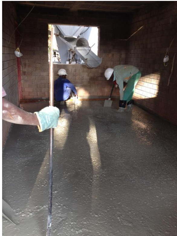
Figure 8-47: The pouring of the floor slabs
