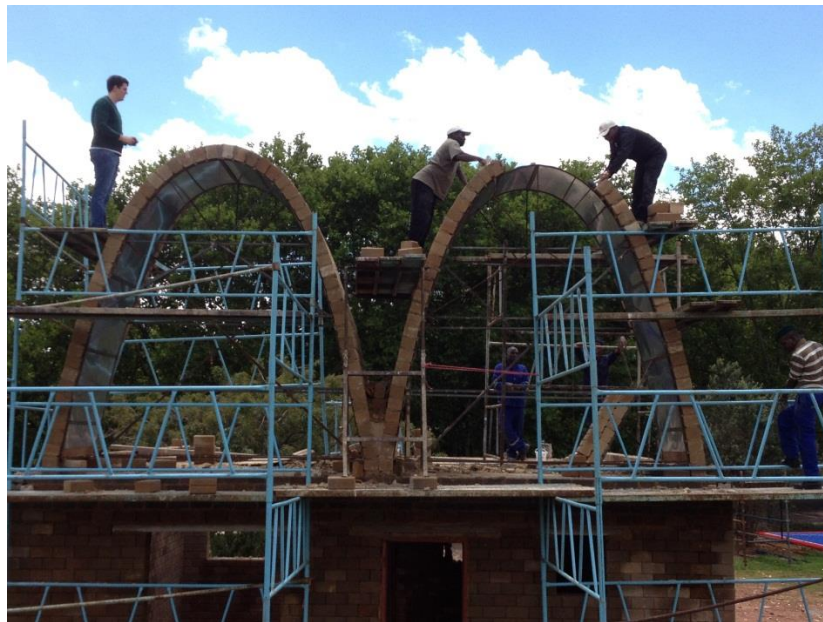
Figure 8-36: Completing the last few layers in the construction of the first section
