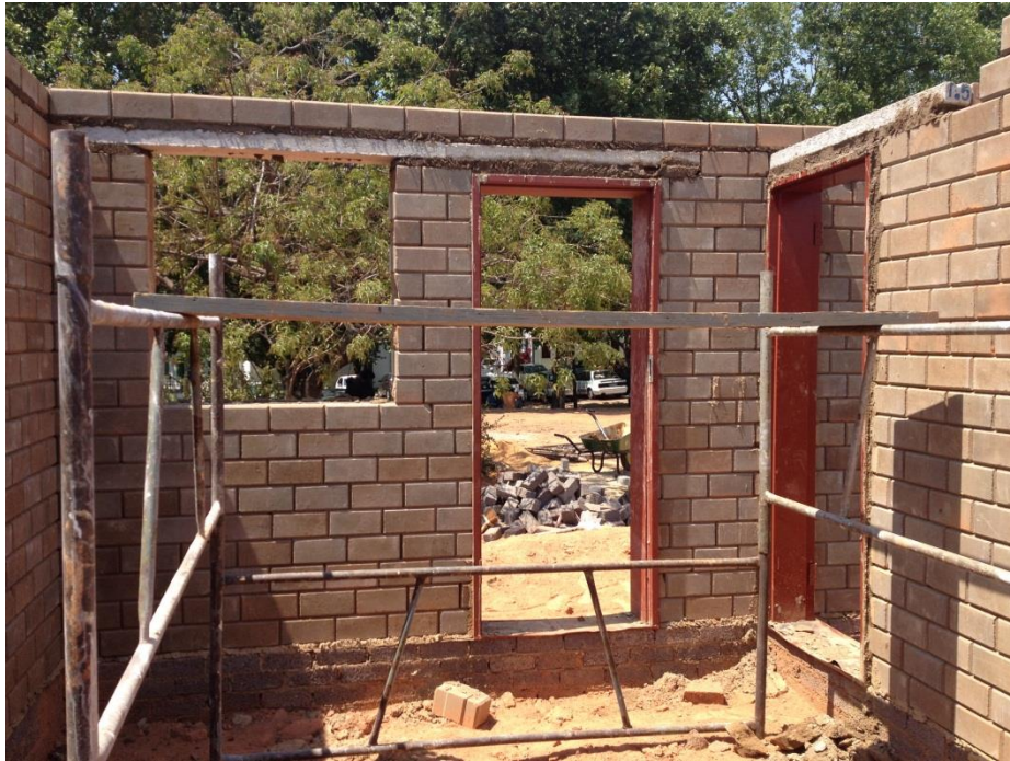
Figure 8-14: Lintels are positioned above all openings to support the bricks above it; the last layer of bricks is mortared in to lock the walls
