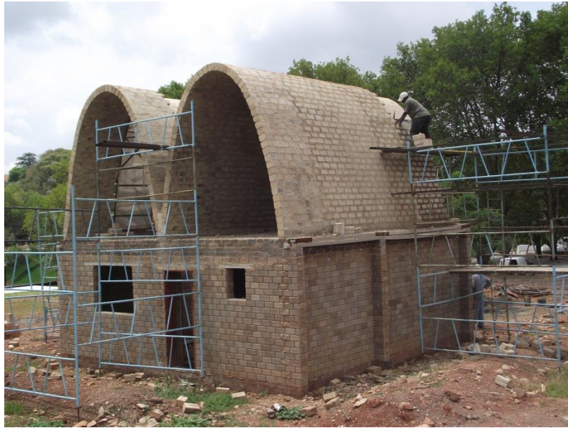
Figure 8-41: Construction of the first vault is almost complete
