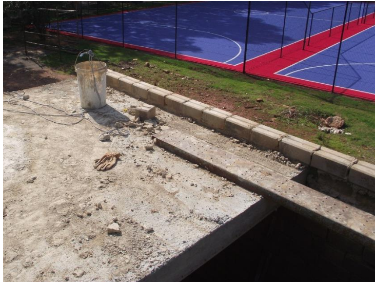
Figure 8-30: The first layer of bricks as at the same level as the slab
