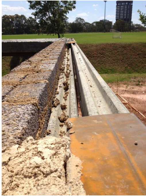
Figure 8-25: The tubes are placed over the lintels and then filled with grout
