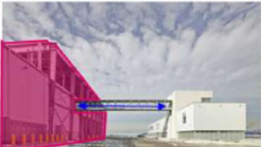
Fig 41: Recycling facility (Author ,2024). base image by (Nikolas k,2014)
