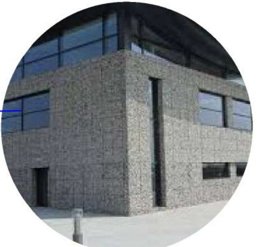
Fig:169. Gabion wall reference image (Unknown,no date)
