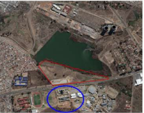
2015: Construction at UJ Commenced. Parking bays on site. Complete Demolition of power station
