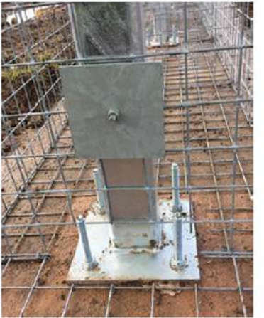
Fig:168. Gabion wall supports,reference image (Unknown,no date)
