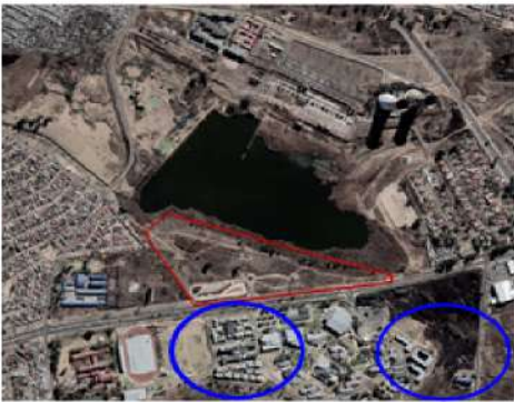
2022: Construction UJ at complete
