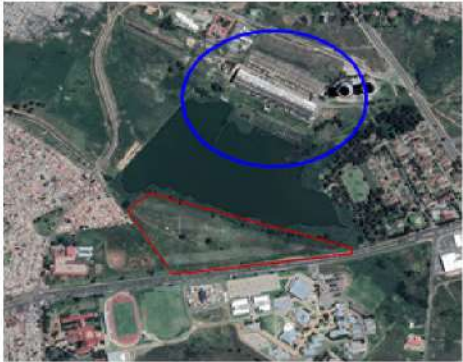
2015: Demolition of the power station commenced.
