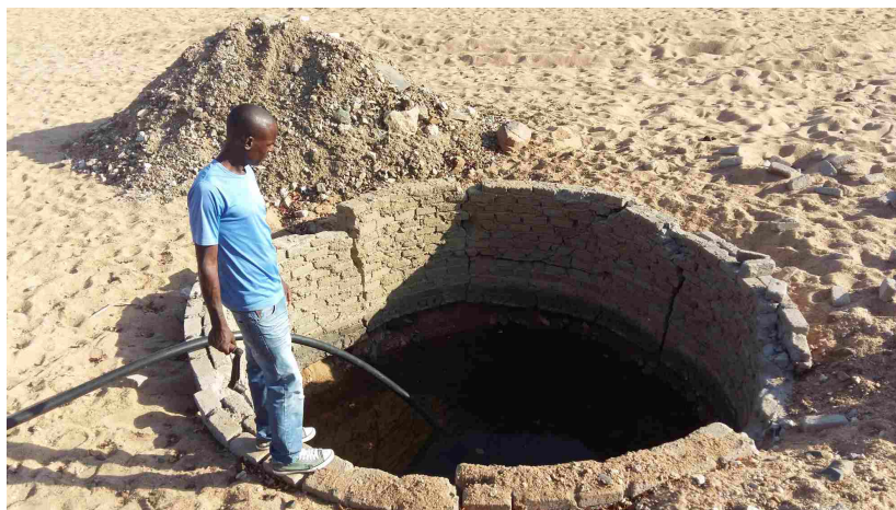
Figure 21: A MFA member inspecting the well he had dug into the dry riverbed bordering his farm, from which he used a diesel pump to extract water for irrigating his crops.
