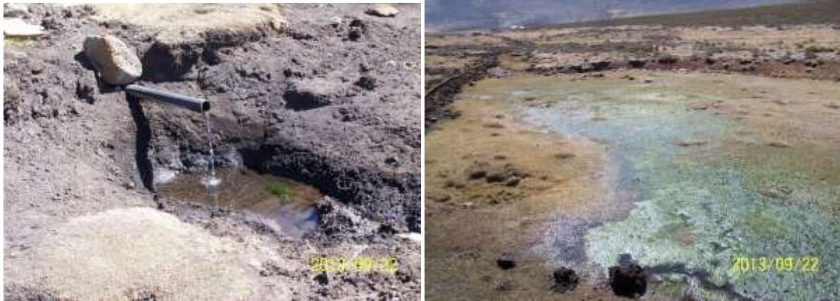
Figure 3.10: PVC pipe inserted into the raised bog, and the resultant standing water with algae.
