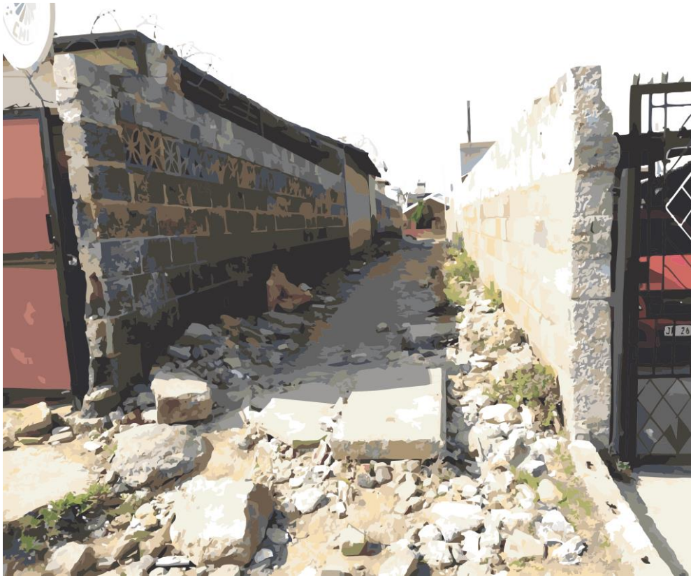
Figure 44: This alleyway between Mahlabathini Street and W Bombo Street (both in the south-west quadrant) is in very poor condition, with high walls, no paving, no lighting and strewn with litter (By Author)
